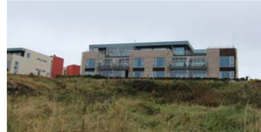
HOUSING BY THE INDUSTRIAL AREA
