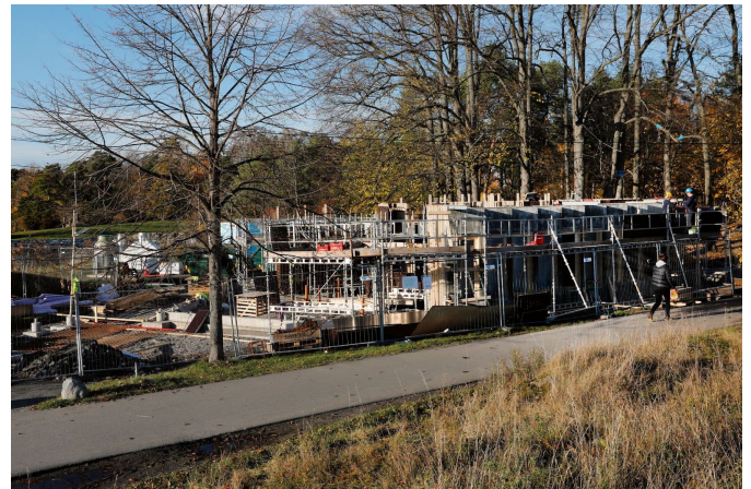
Picture 9: Building the service building. Signe Dons. 2020
