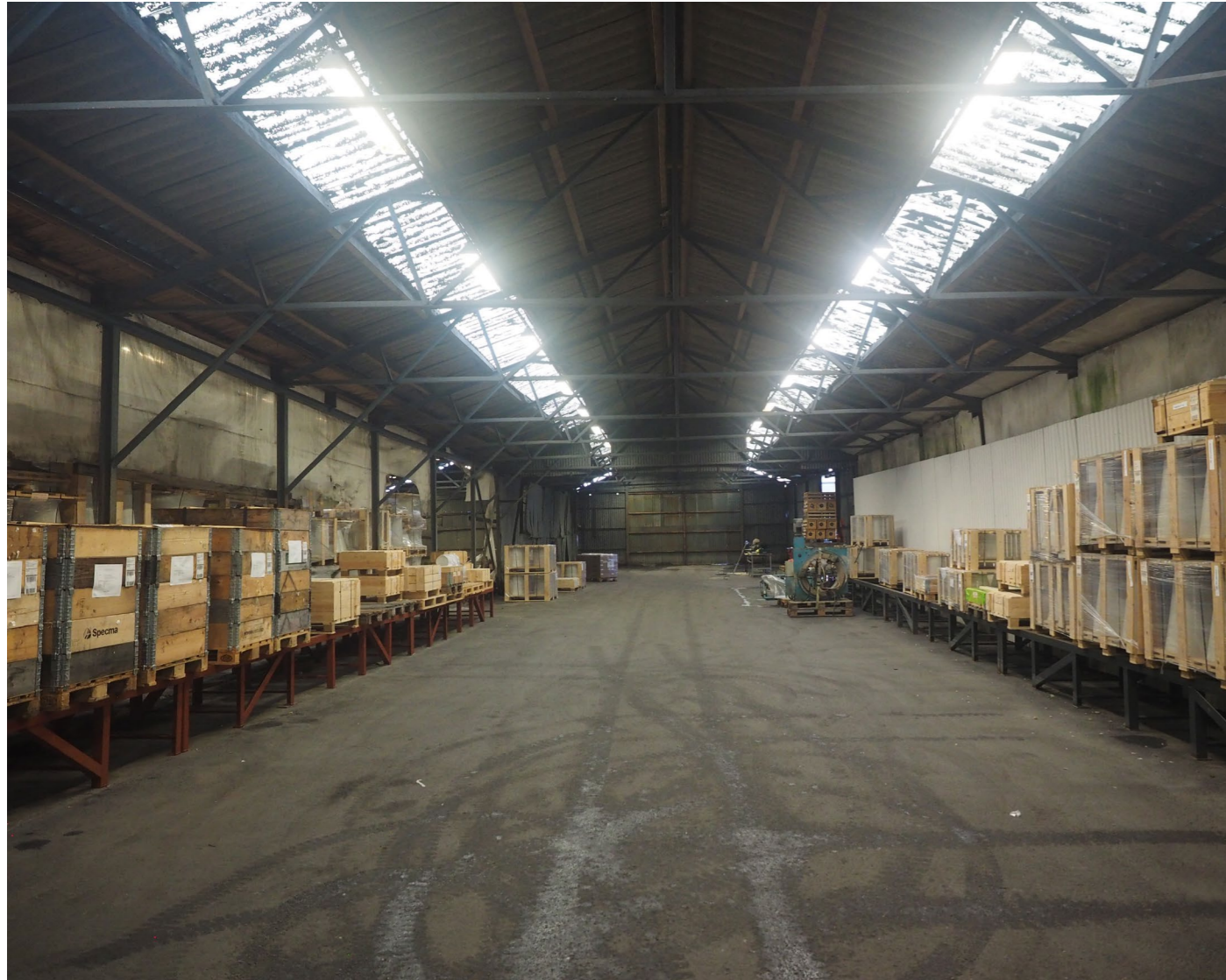
Existing storage shed
