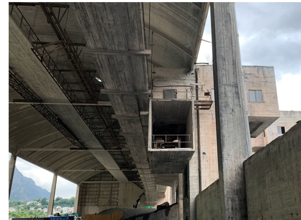
Current state of the structure, facing south. August 2020.
