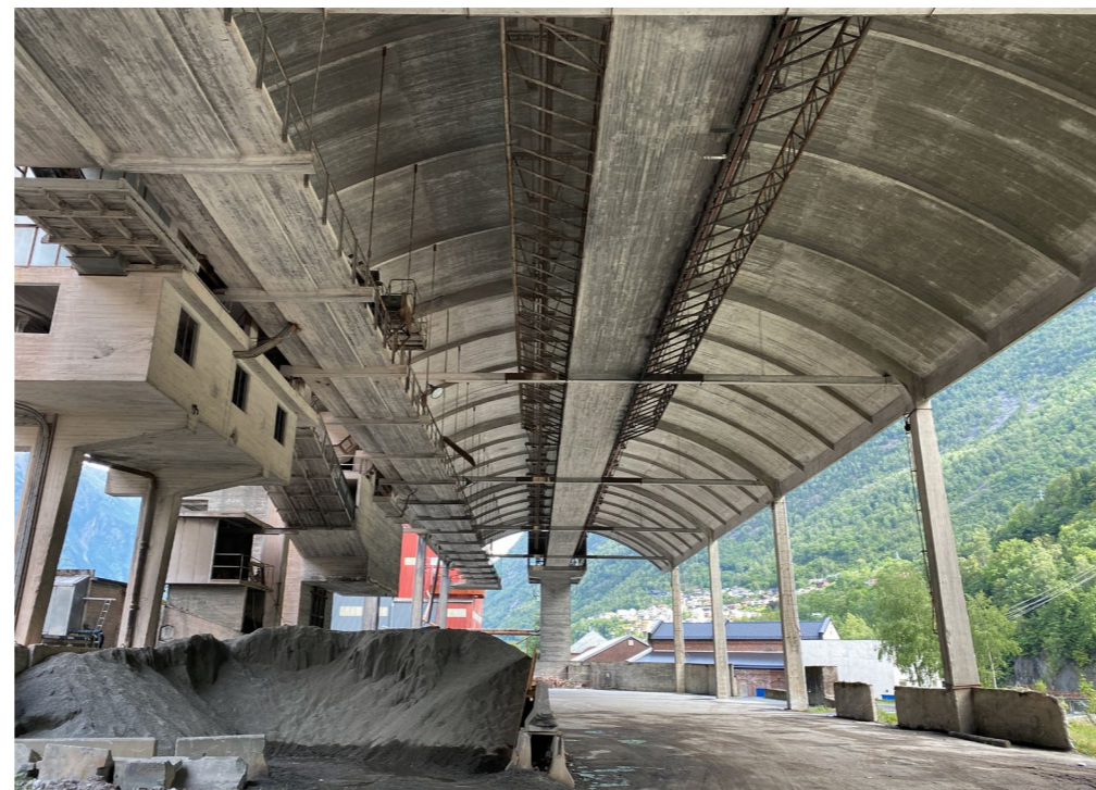
Current state of the structure, facing north. August 2020.
