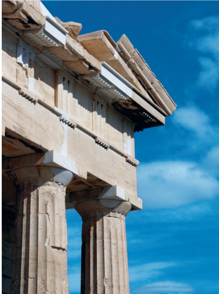
1 Tasos Tanoulas, Anastelosis of the east front of Propylaia, Acropolis, Athens, 1990–2010. New blocks of Pentelic marble are slightly lighter than the original ones.
