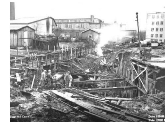
The piping the stream in 1950s and growing city brot significant change. The place became industrial area. Those 2 streams were connected much Northern than the original trace used to be so that Hovind Valley became disconnected from its main water source and now its fuel only with its own micro catchment.
