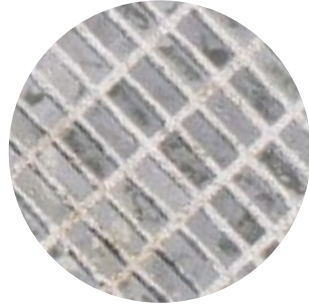
Pavers 75% density with pebbles
