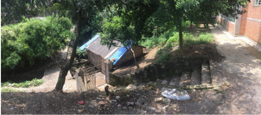
Figure 5.27: The site for a pedestrian bridge. The photo was taken on September 2, 2016. (Source: Author)
