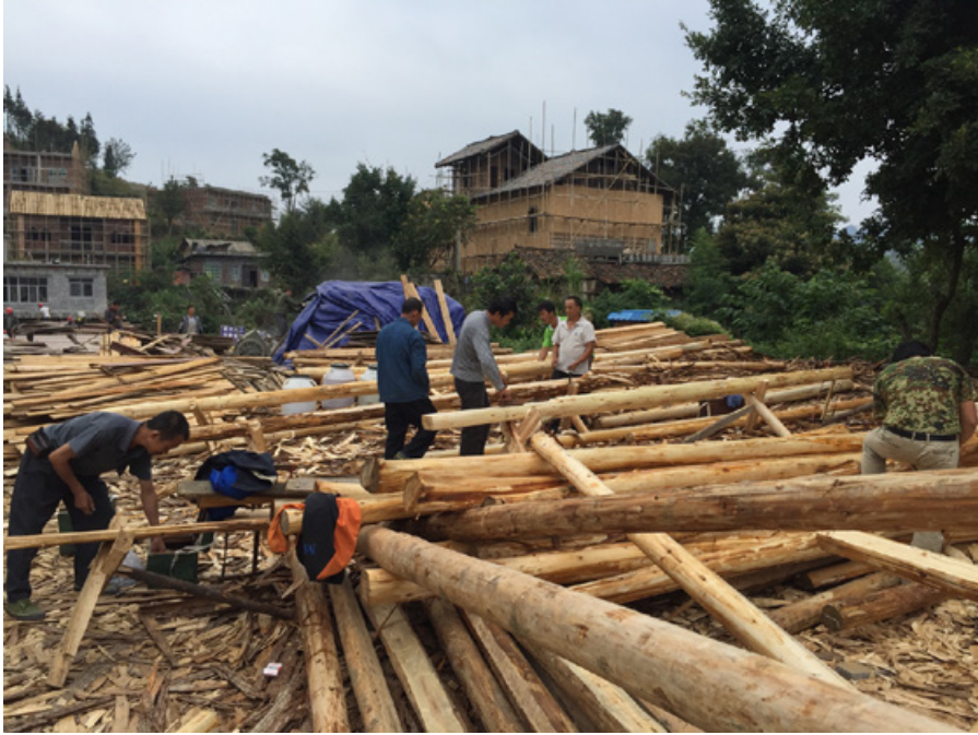
Figure 5.37: Skilled craftsmen perform rough processing on the imported wood materials. The photo was taken on August 16, 2016. (Source: Author)
