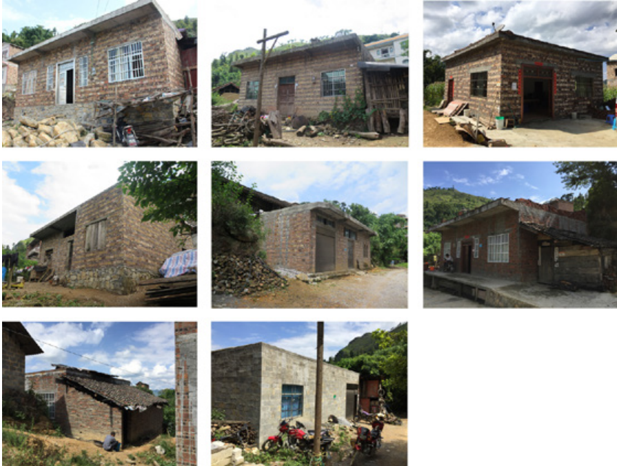
Figure 5.42: The expert architects devised a new facade treatment that mixed mud, wire meshes, cement mortar, and gravel. The photo was taken on September 5, 2016. (Source: Author)
