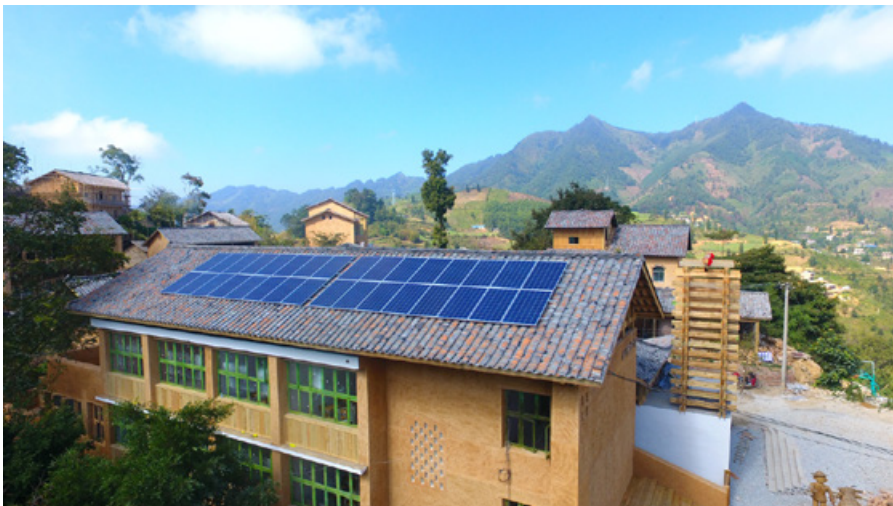
Figure 5.76: Solar panels were installed on the rooftop of the school building. The photo was taken on November 18, 2016. (Source: Author)
