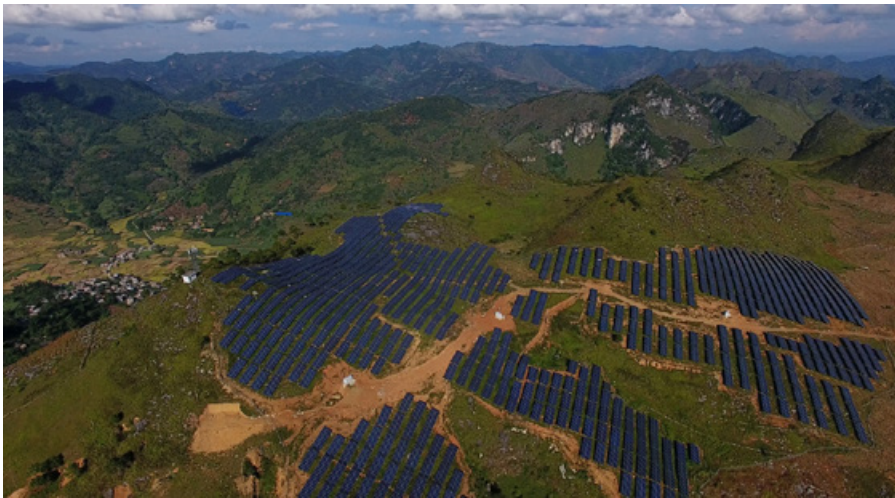
Figure 5.89: The power company constructed the solar panel matrix on the south-facing slope of Bugong Mountain. The photo was taken on October 4, 2017. (Source: Author)
