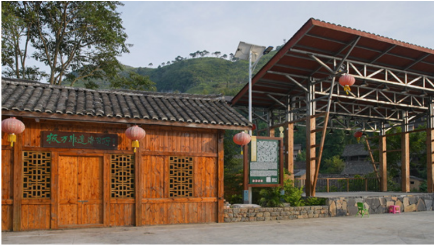
Figure 5.31: The completed rehearsal room and performance stage. The photo was taken on August 5, 2021. (Source: China Central Television, Yu Lin, and Zhuang Nan)
