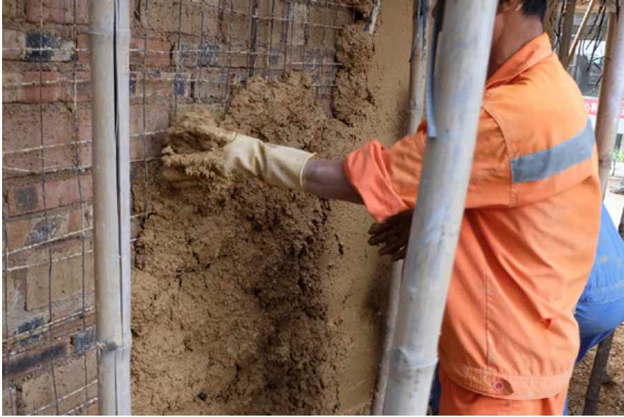
Figure 5.42: The expert architects devised a new facade treatment that mixed mud, wire meshes, cement mortar, and gravel. The photo was taken on September 5, 2016. (Source: Author)
