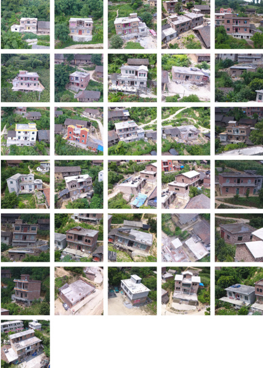
Figure 5.11: There are 31 newly built prefabricated concrete and brick buildings, 21 of which are two-story dwellings. (Source: Author)
