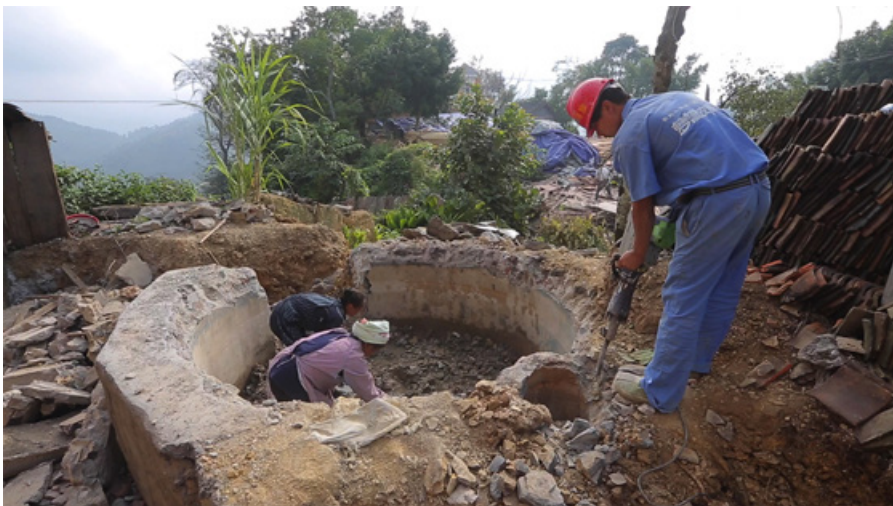
Figure 5.66: Architects took advantage of the abandoned biogas tank and transformed it into a new kiln. The photo was taken on September 26, 2016. (Source: Author)
