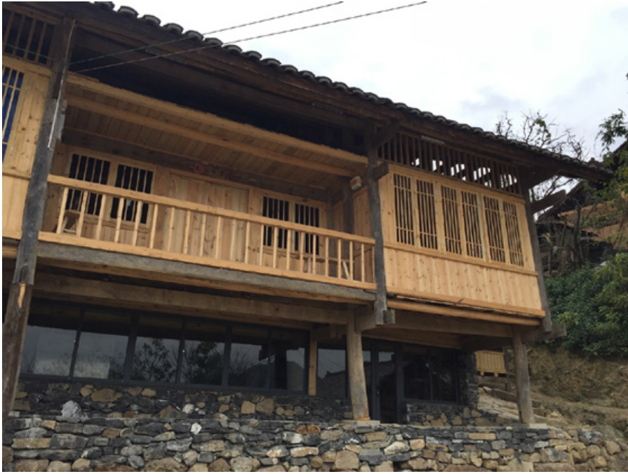
Figure 5.73: The lower semi-outdoor space for livestock was transformed into a kitchen. The photo was taken on November 10, 2016. (Source: Author)
