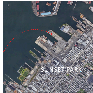
...and into the onshore substation
