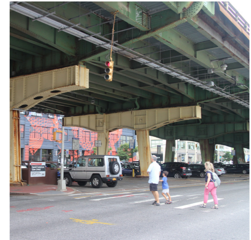
Pedestrian crossing under Gowanus Expressway
