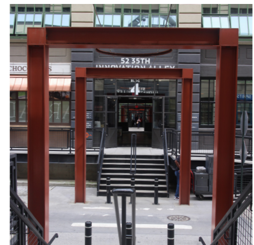
Connection crossing the Industry City buildings
