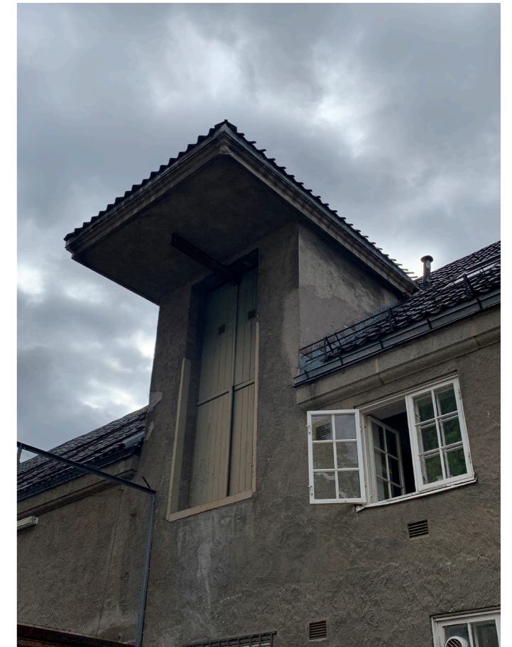
The other hayloft on the other roof.
