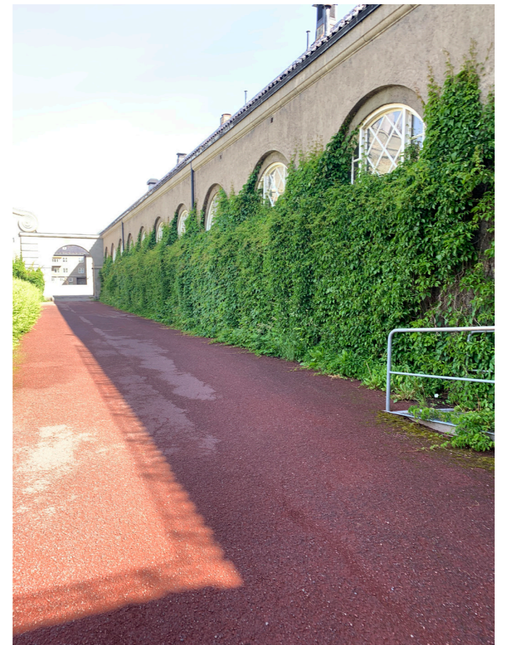
the south-west facade facing the courtyard
