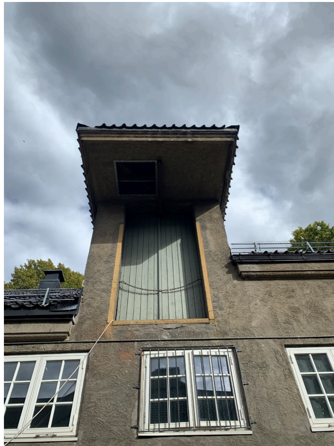
The eave change height when it meets the hayloft.
