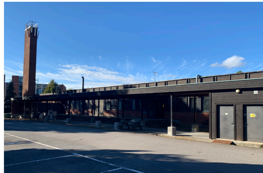
A "mønstringstripe", for horses to walk back and forth, covered with roof.
