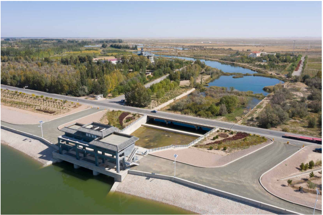
Fig. 2.1: The Hongyashan Reservoir in Minqin County has been built to hold back the limited water sources and allow for a controlled supply of farms in the lower, exposed reaches of the Shiyang River watershed; September 2019.
