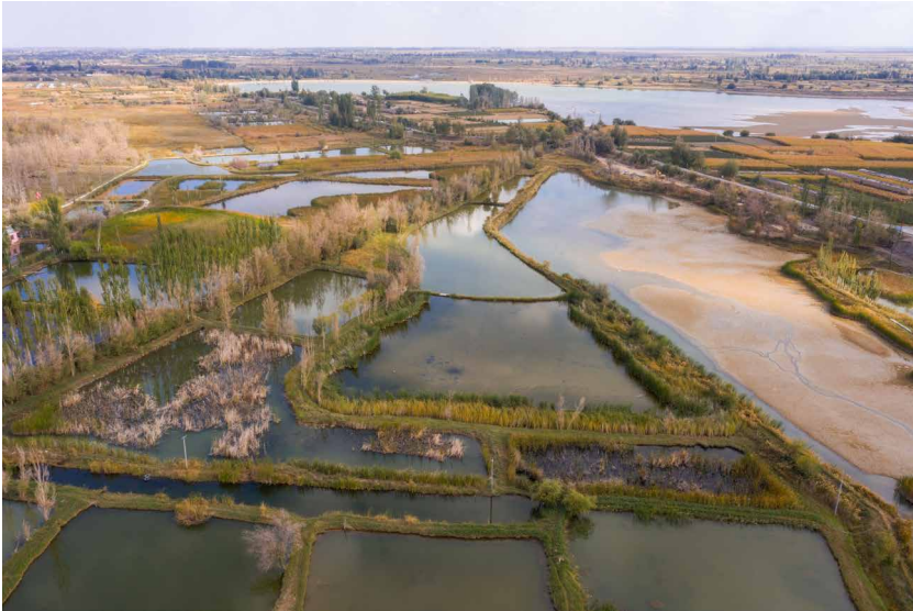
Fig. 7.1: North of Jiuquan, a landscape has been created combining heavy engineering with traditional land uses and nature-based solutions. The dynamic, small-grained, and multilayered ecosystem provides rich habitats, integrating various waterbodies, wetlands, and vegetation patterns, as well as housing, tourism, farming, livestock, and fishing; October, 2019. (above and following pages)
