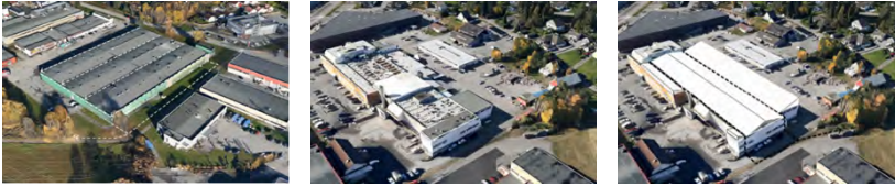
Figure 91: The conversion of internal to external drainage entails interventions to the existing buildings. Ill: Author.
