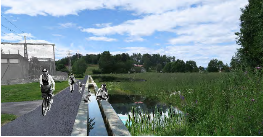
Figure 82: Illustration of Kjørbekk at the level of the power transformer. Here, the water is controlled in an elevated channel to avoid the need to change the position of the high-tension installations that are found underground close to the surface. Ill: Worksonland.
