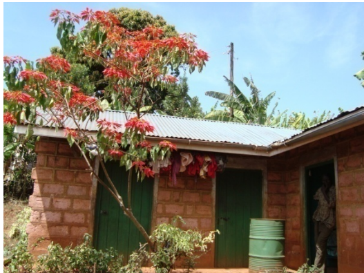
Fig. 6.12 The first fired blocks building in the study area built in 1974. (Source: Author 2009)
