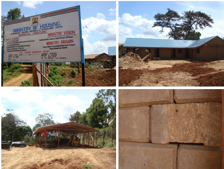
Fig. 4.52 Appropriate Building Technology Centre in Mukurwe-ini, Nyeri. (Source: Author, 2009)
