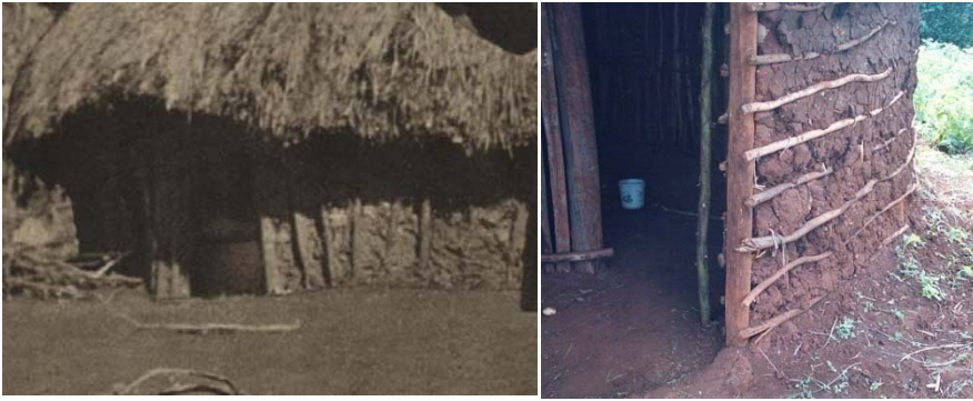
Fig 3.5 Examples of mud wall constructions.
