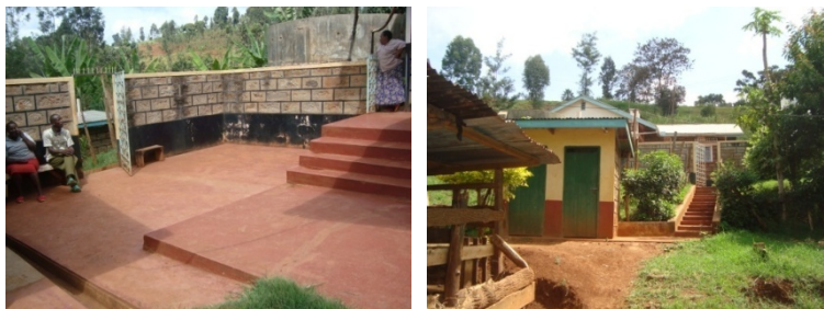
Fig. 5.54 Control of levels in the paved Nja (Source: Author, 2009)
