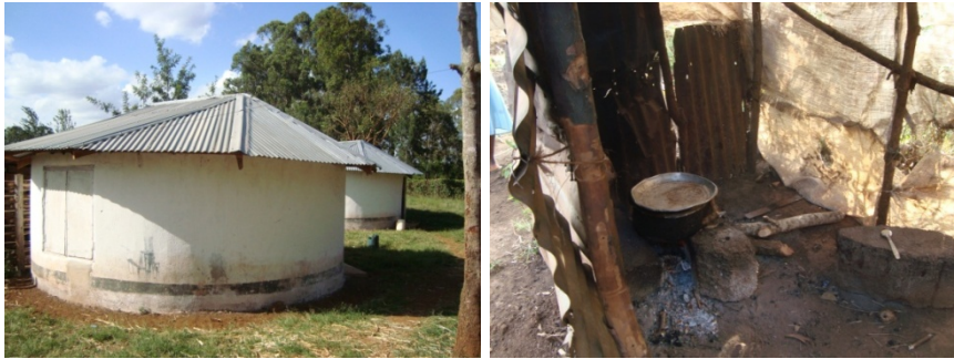
Fig 4.30 More Former Settler Coffee Estates Workers Housing in Thika (Source: Author, 2010)
