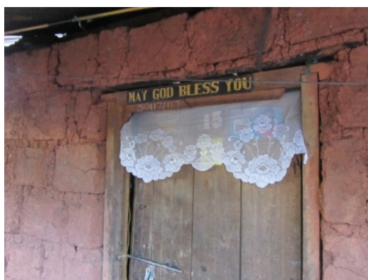
Fig. 6.19 A more elaborate construction with the blocks joined with cement and on two courses of quarry stone foundation. The floor will be cemented while the roof will sit on a reinforced concrete lintel. (Source: Author 2012)
