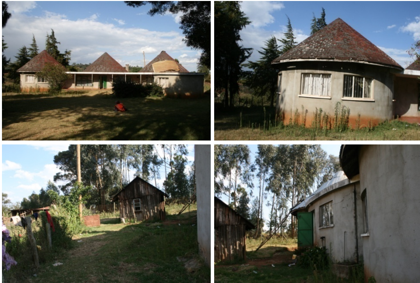
Fig. 4.55 Ngugi wa Thiong'o House in Limuru (Source: Author, 2009)
