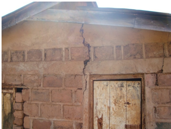
Fig. 6.20 Mud blocks made to look like stonework with a fake reinforced concrete lintel. In time, depending on the stability of the foundation, big cracks sometimes appear giving the game away. (Source: Author 2009)
