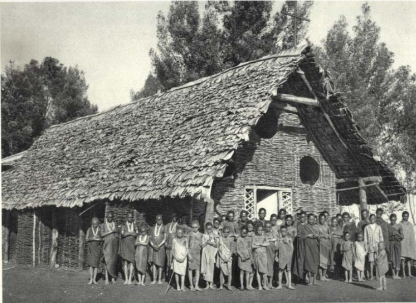
Fig 4.9. Early Church built in traditional gikonjo style. (Source: Cagnolo, 1933) The roof was beautifully done in banana bark.
