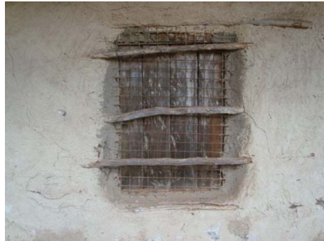
Fig. 5.75 Mud and wattle wall structure well exposed in collapsing wall. This is what happens to an unused mud house within a span of seven years. (Source: Author, 2009)
