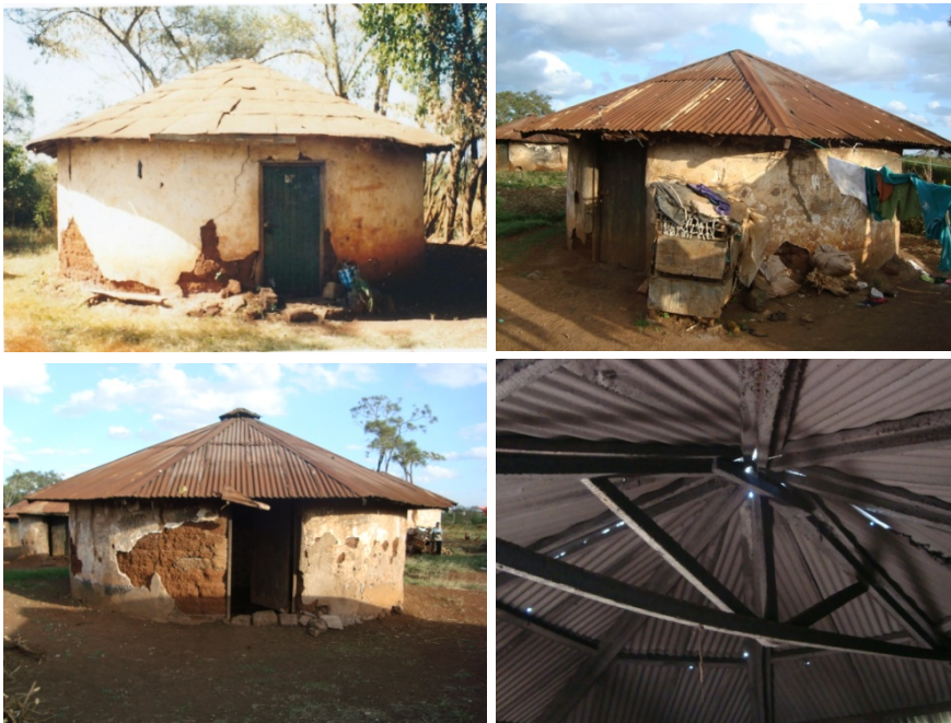
Fig. 4.32 Coffee estates workers housing in Thika. (Source: Author, 2010)
