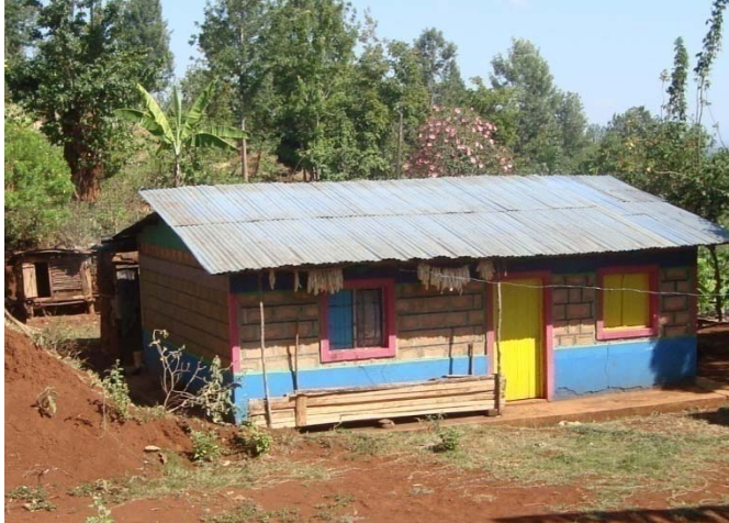
Fig. 6.22 A thoughtful finishing of the mud blocks protecting the critical areas with cement plaster. (Source: Author 2009)
