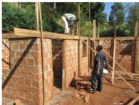
Fig. 6.19 A more elaborate construction with the blocks joined with cement and on two courses of quarry stone foundation. The floor will be cemented while the roof will sit on a reinforced concrete lintel. (Source: Author 2012)
