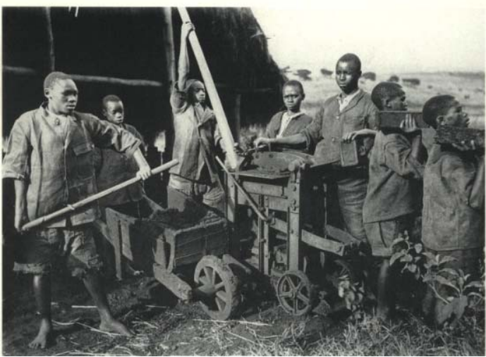
Fig 4.10 Students in an early missionary construction class making mud blocks. (Source: Rigamonti, 2001)
