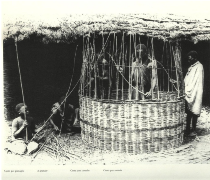
Fig 3.21 Constructing a granary. (Source: Rigamonti 2001)
