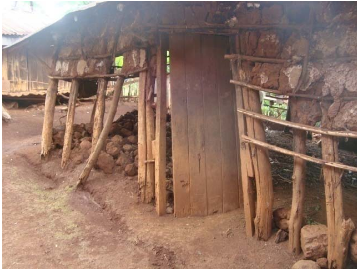
Fig. 5.75 Mud and wattle wall structure well exposed in collapsing wall. This is what happens to an unused mud house within a span of seven years. (Source: Author, 2009)
