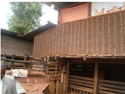
Fig. 5.68 Construction of the goathouse.
