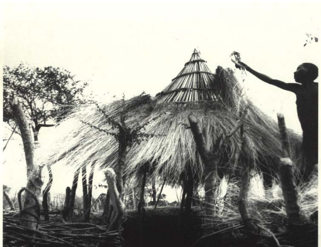
Fig. 3:23 Construction of a granary roof. (Source: Rigamonti 2001)
