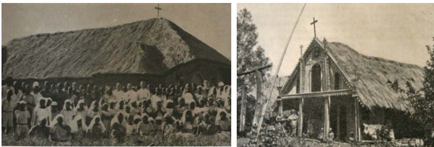
Fig 4.11 Examples of early Consolata Mission Architecture (Source: Mathew, 1952) Top left: Merely titled: a primitive church in Kikuyuland. Grass thatch roofing of the 1900s Top right: Church at Karima. Grass thatch roof and galvanized sheets façade. (Karima mission founded 1904)
