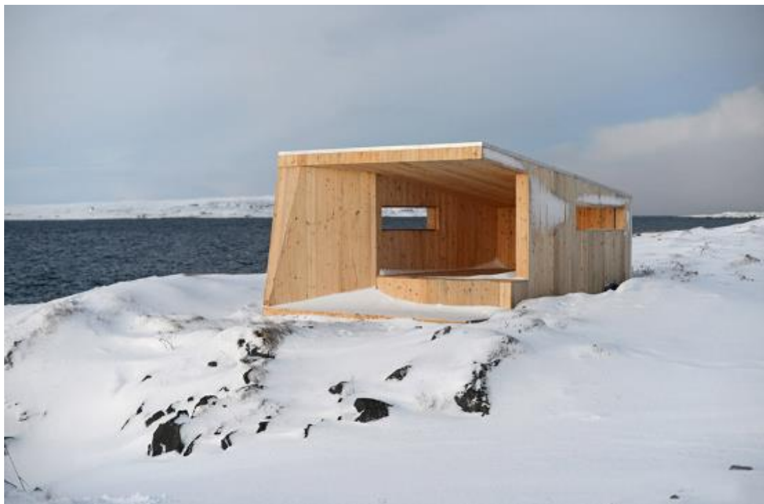
Figure 2. The Steilnes bird hide (Vardø, Norway, 2012) is carefully located in relation to view, microclimate and bird behaviour. Design: Biotope (photo: T. Amundsen).
