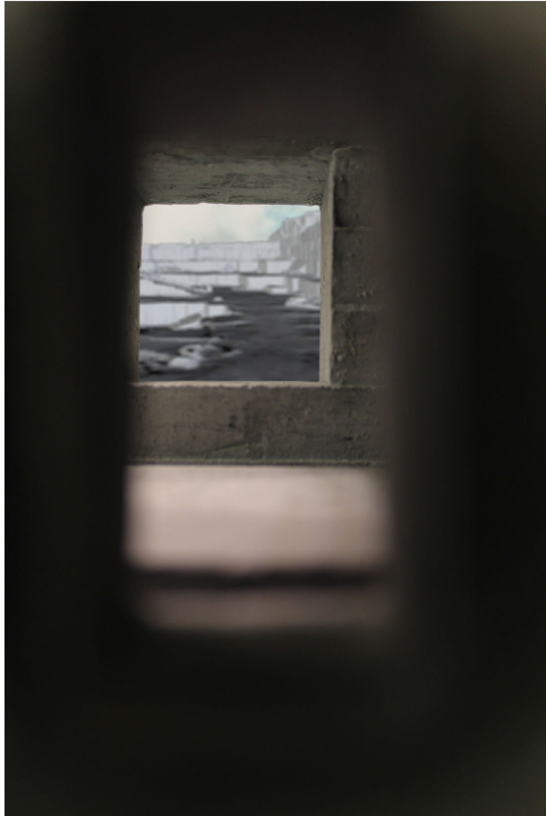
Entering the water dam space
