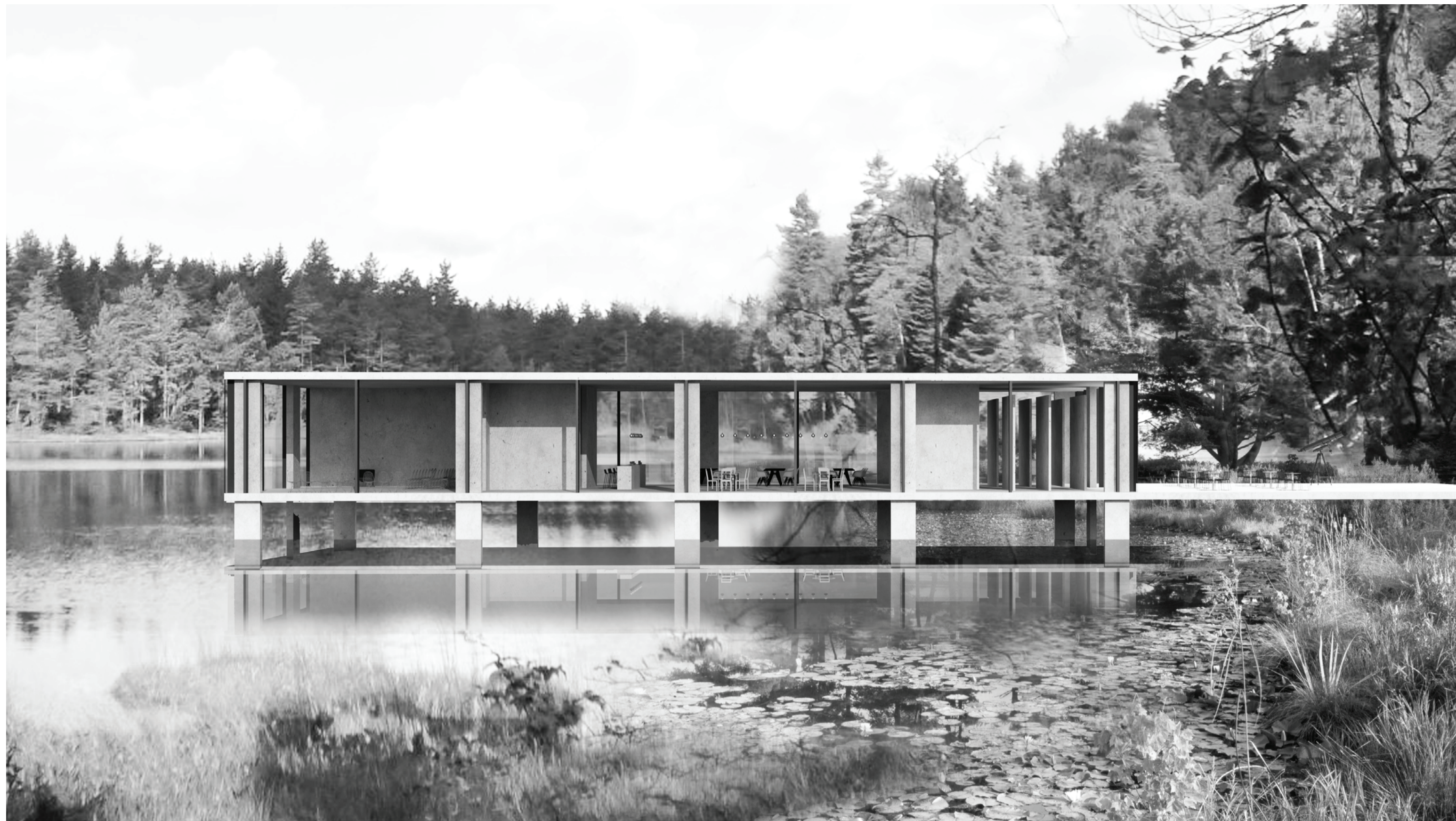
Visitor center exterior view
