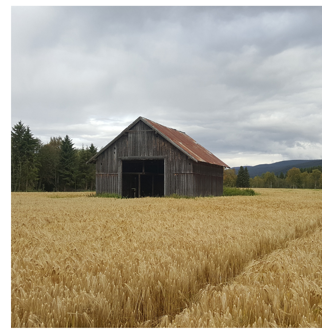
Barn located in Ekeberg. Older barn with high quality construction using the 'toll' technique. The structure is sturdy, durable, and would need some attention. The barn consists of three smaller sections with an old storage. Project: 2247.
