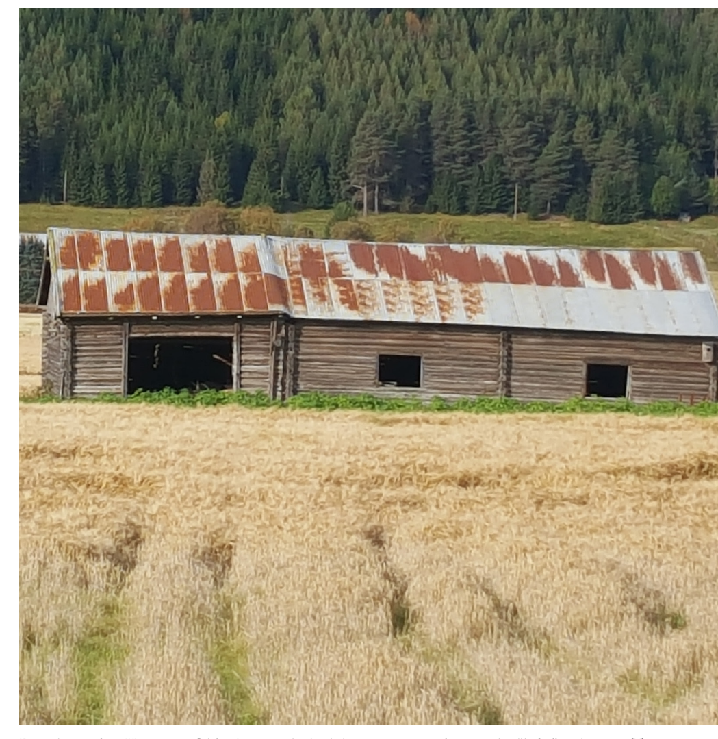
Barn located in Ekeberg. Older barn with high quality construction using the 'toll' technique. The structure is sturdy, durable, and would need some attention. The barn consists of three smaller sections with an old storage. Project: 2247.
