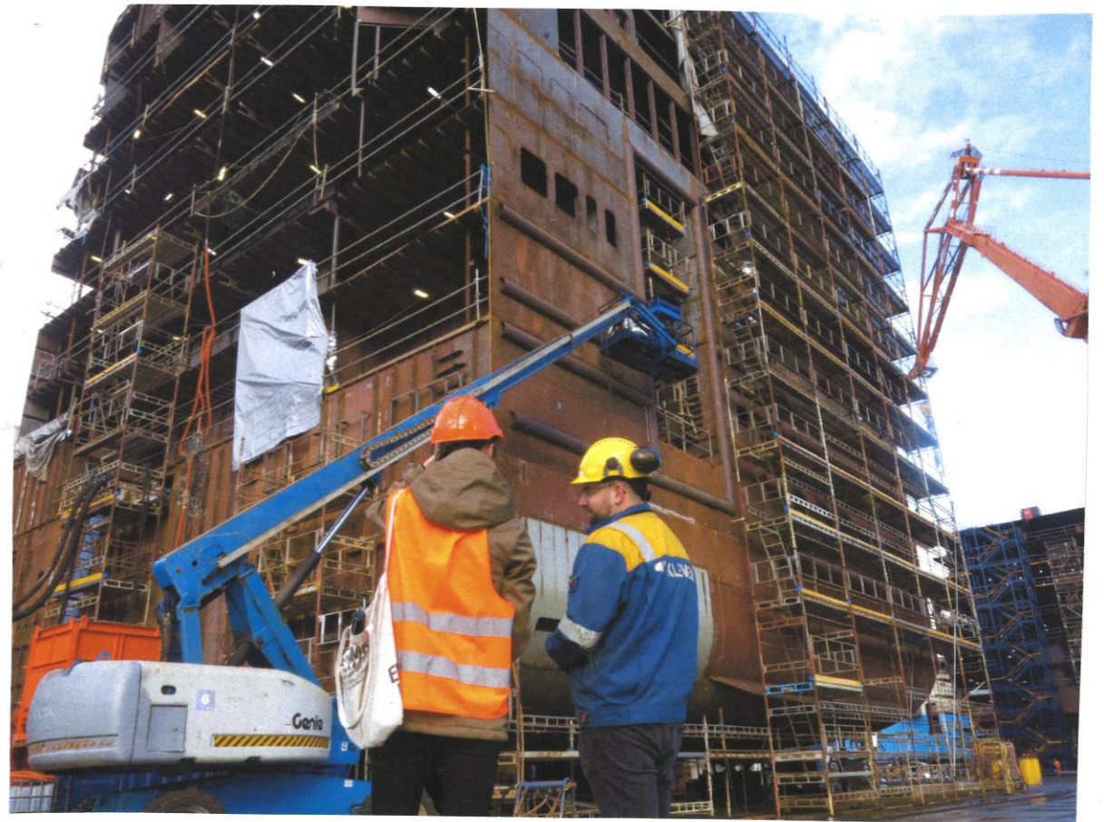
THIS BLOCK IS APPROX. 24x24M AND 11 DECKS HIGH
