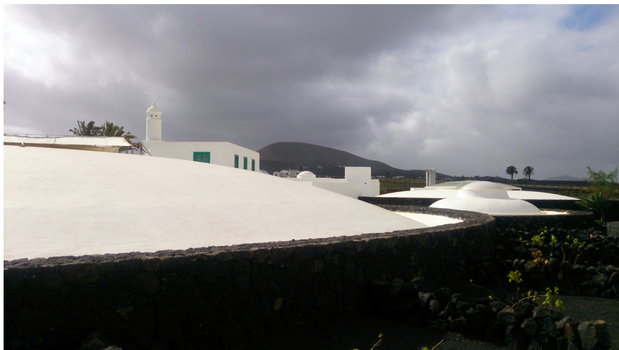
Figure 10: César Manrique's architecture refers to local tradition as well as creative expression, reflecting the dramatic volcanic landscape of Lanzarote (Casa-museo del Campesino). (Photo: Birger Sevaldson.)
