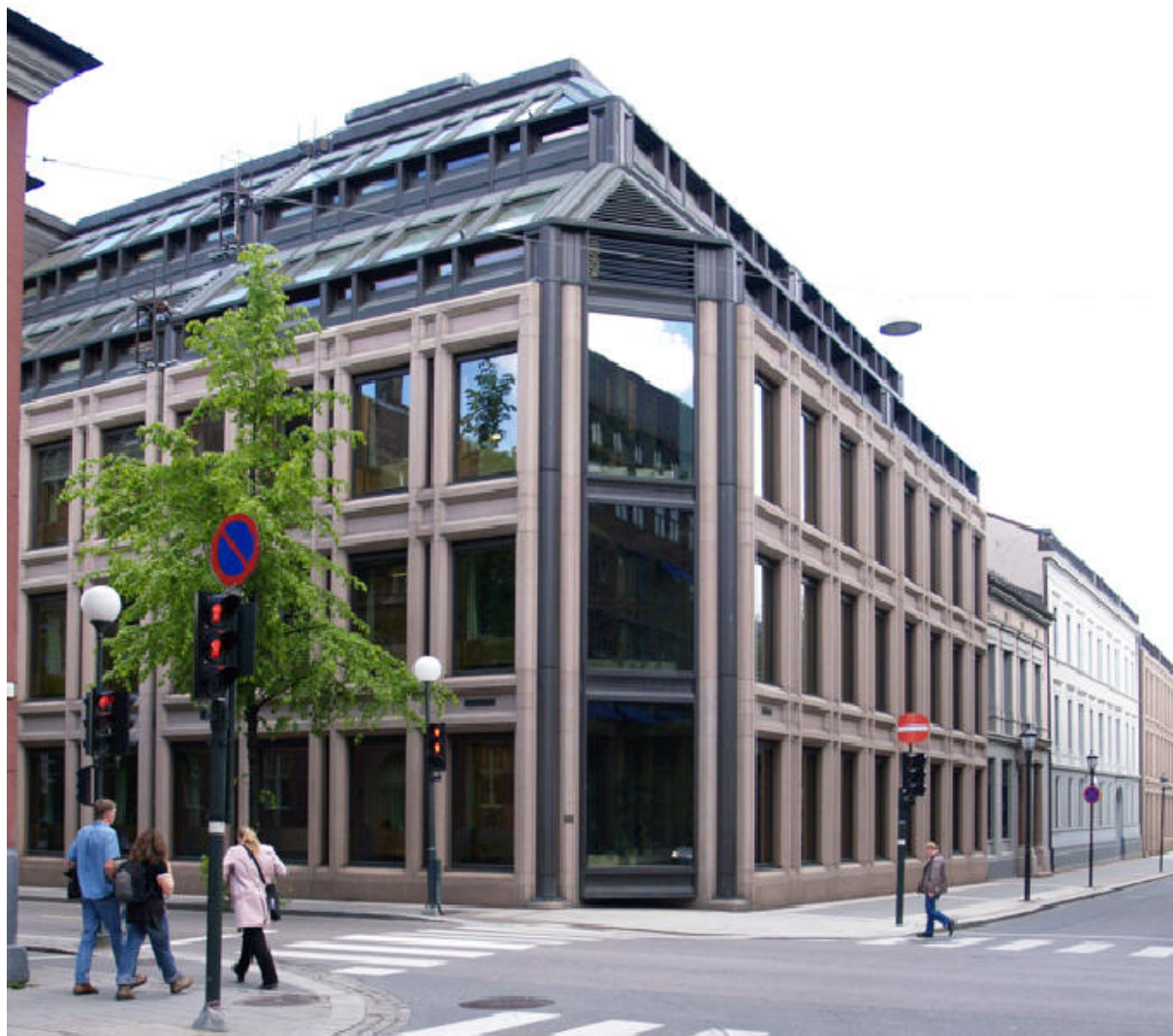
Figure 8: National Bank of Norway (1986). An example of holistic design degenerated to formalism. The same profile, most notably in the horizontal section of the corner of the building, is repeated at different scales throughout the building. Architects: Lund & Slaatto A/S. (Photo: Wikimedia Commons.)
