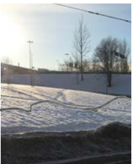
open gap along tram line
