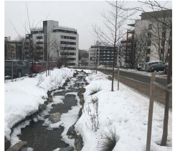
In the winter conditions, little vegetation filters effusions from either the car park or road.
