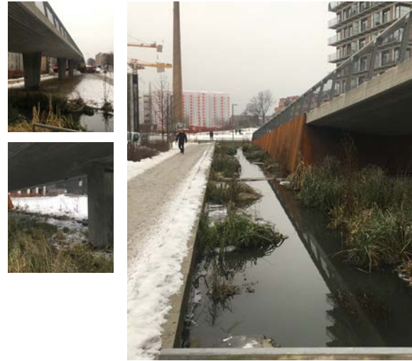
Water body expanded under the bridge and fully on the other end. The vegetation is not dormant but green and saturated.
