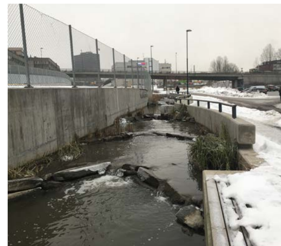
In winter, the neighbor car park places plowed snow in a heap. The effusions may run directly into the stream. The adjacent sidewalk is fully iced, showing that water is melting and moving along the route.
