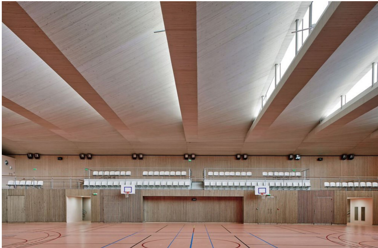
Skylight from north facing clerestory windows
