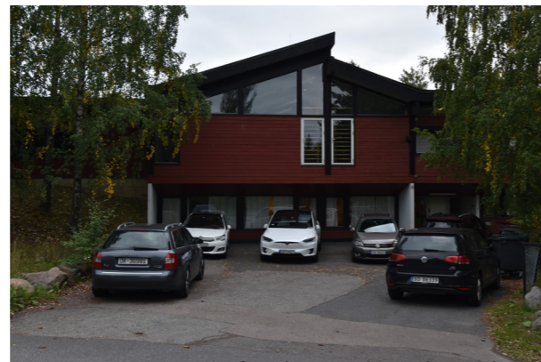
2.3 - facade towards north- south axis
