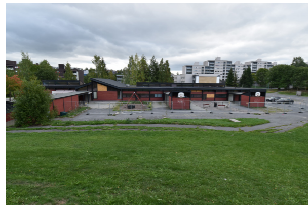
2.1 - existing building on site
