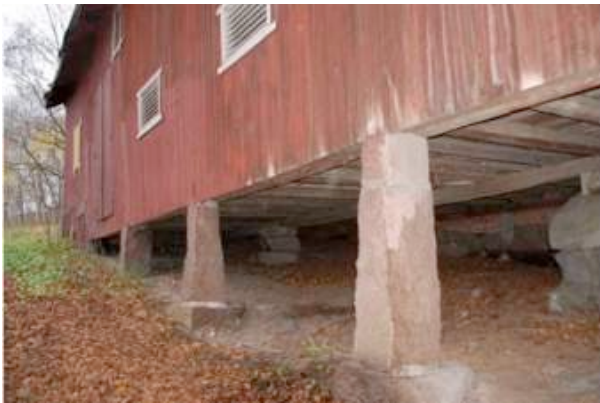
The foundation pillars are in perfect condition.
