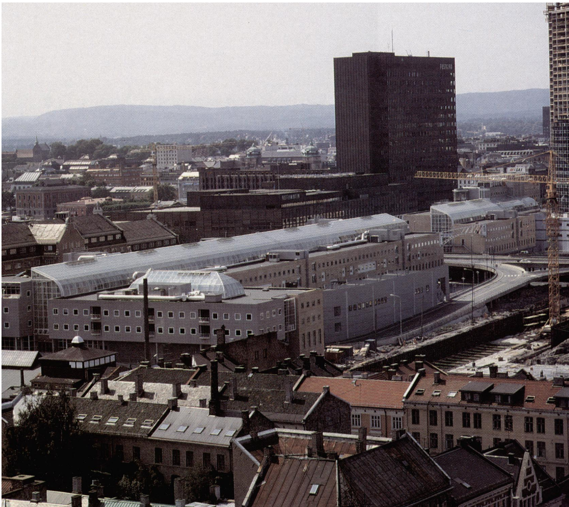
Clockwise from top: south facade; east facade; north facade
