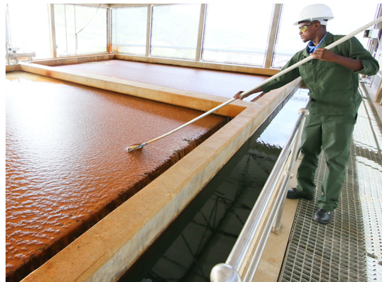
6. Wingoc employee inspecting effluent at the New Goreangab Water Reclamation Plant
