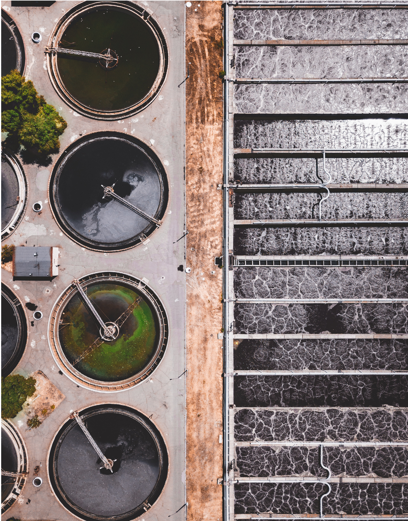
3. Advanced wastewater treatment plant in USA
