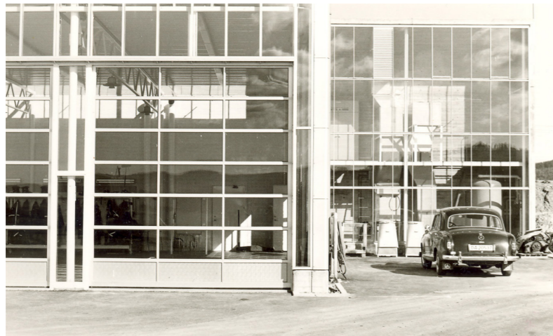
(Kvalviknes 1970) Steel structures inside, exposed through car gates
