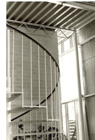
Detailed steel structures inside
