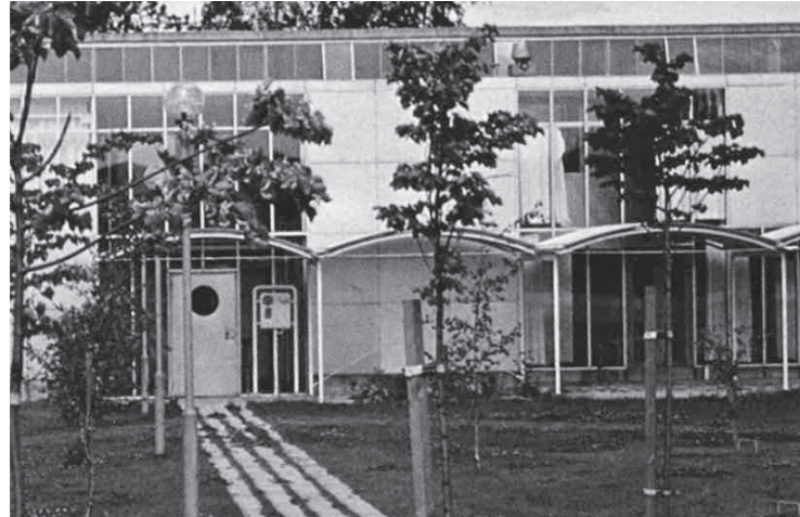
(Grønvold 1984: s. 423) Main facade clad in aluminum plates, as well as exterior steel structures maintain a technical "touch"
