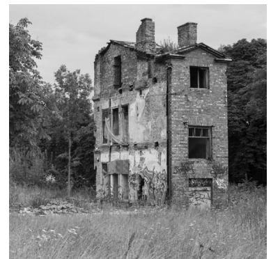
Remains of a burned down Tallinn style house at Kopli Liinid in northern Tallinn. The central staircase was built in brick, complying with fire-safety regulations at the time.
