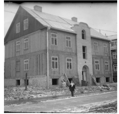
A Tallinn style house at Ristiku street 15. In this image the building has yet to receive its paneling.
