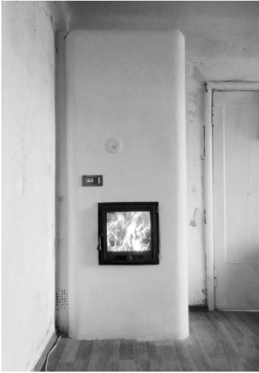
A newly modernized masonry stove, equipped with a digital thermometer.
