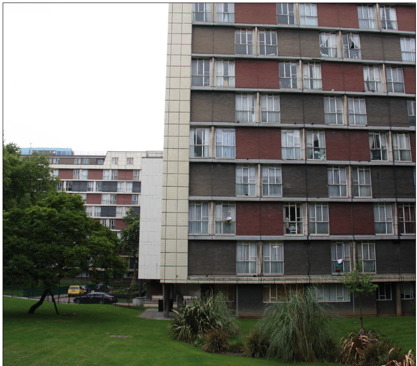
Figure 4. Infilled pilotis at Denys Lasdun's Hallfield Estate, 1951–58. Photo: Tom Davies, 2012
