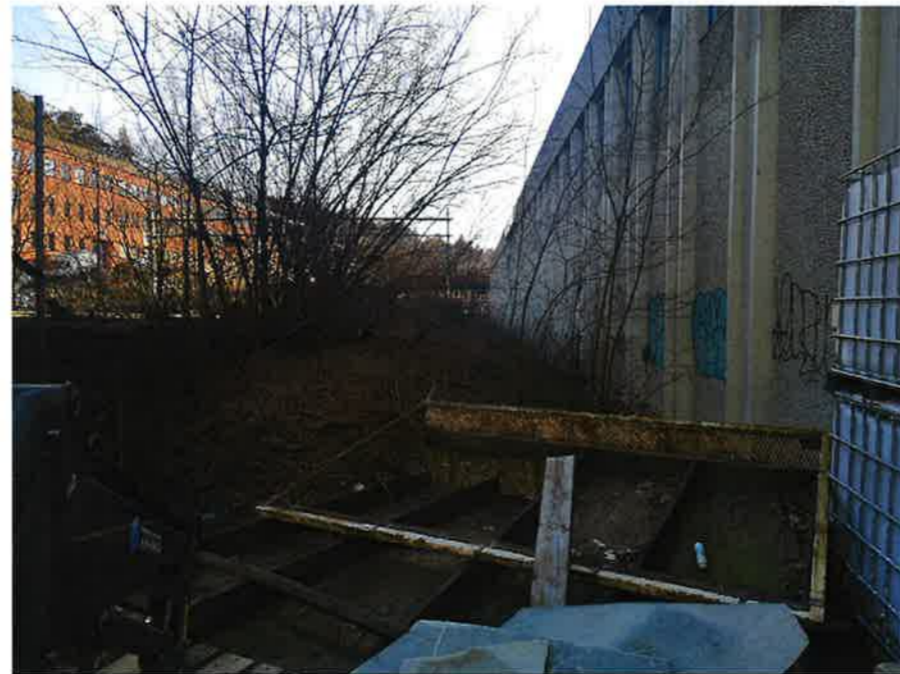
26. The storage building placed on top of the river
