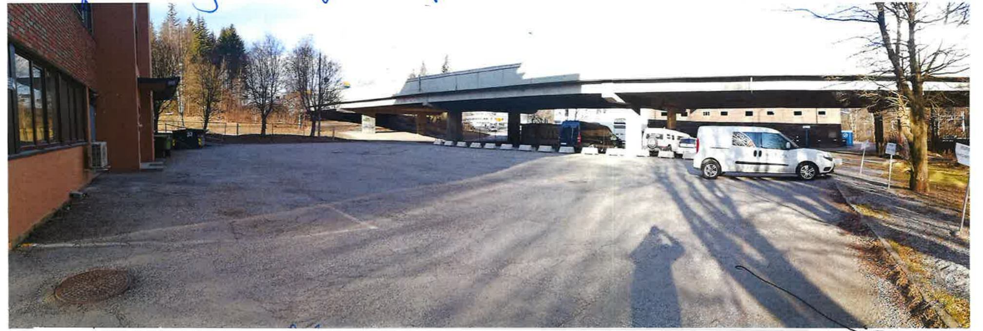
6. left office building, right elevated highway and Kristiania Teglverk. The parking lot between the buildings is partly used.
