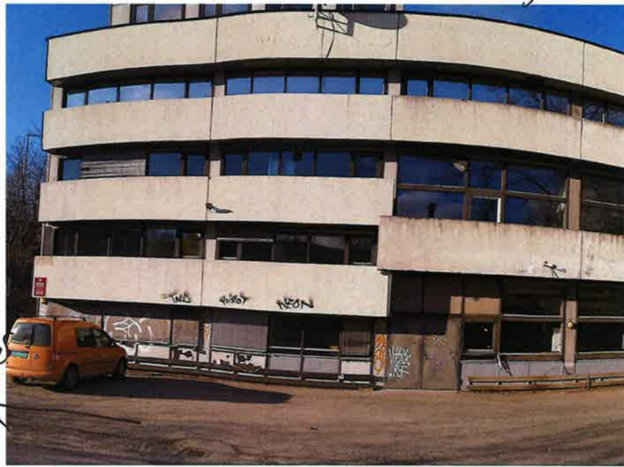
3. Abandoned building, not used parking lot in front.
