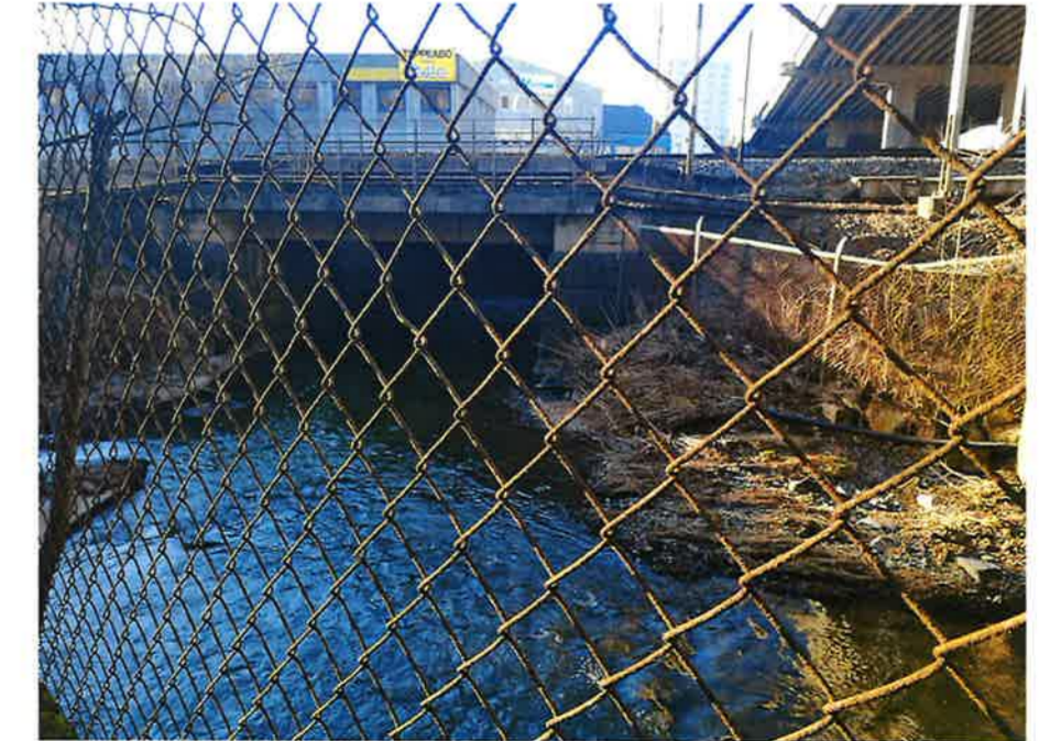
32. Can the path D10 get an alternative route under the bridge?
