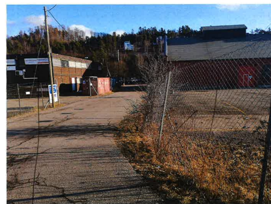
17. temporarily bricked little used asphalt surface zinc white factory
