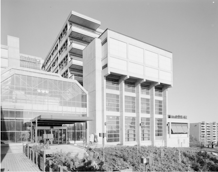
13. Romsås Centre. Photograph by Teigens fotoatelier, 1977. DEXTRA Photo, Norsk Teknisk Museum. Licenced under CC BY.
