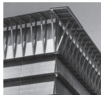
Ricola Storage Building by Herzog & de Meuron, 1987. The beautiful façade of fiber cement sheets covers a standard sandwich element wall.
