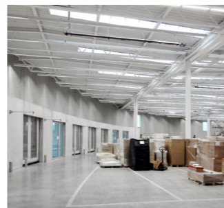
Factory Building on the Vitra Campus by SANAA, 2012. Circular plan, but with a load bearing system following an orthogonal grid.
