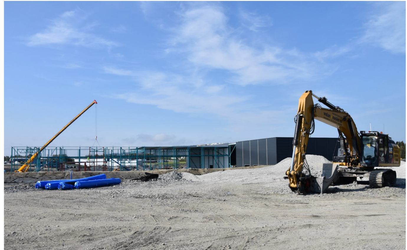
The Hydroscand construction site at Lindeberg near Oslo. August 2019
