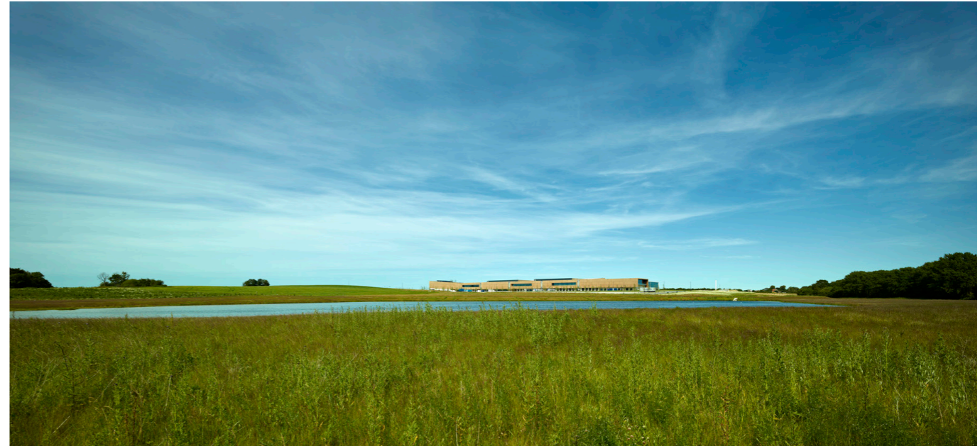
Bestseller Logistics Centre North by C.F.Møller Architects
