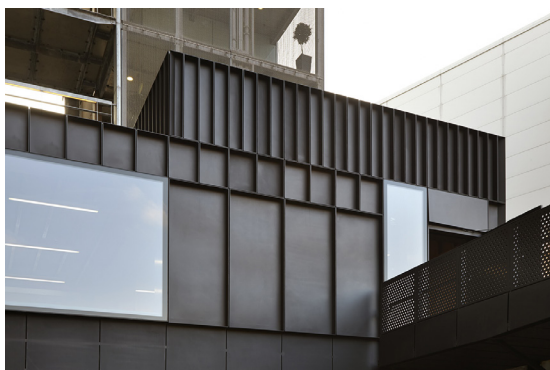
Project: Shepherds Building Site: London, UK Year: 2013 Area: 10,000 m 2
