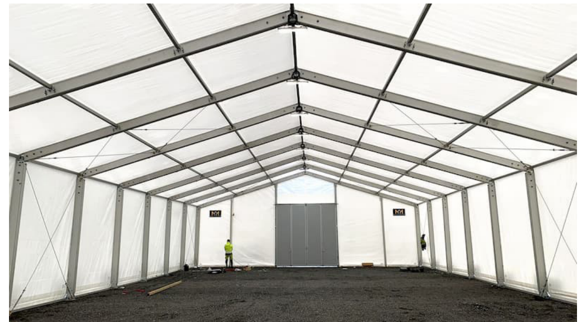
Typical tent used for covering construction
