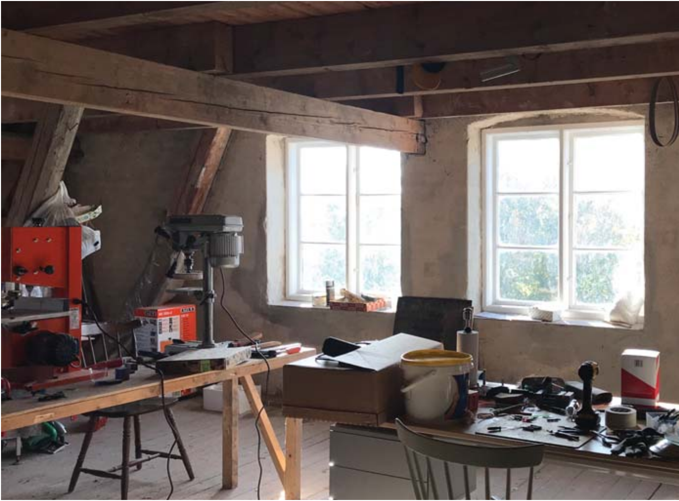
Photo of the third floor in the southern part. Note the big dimension of the timber construction.
