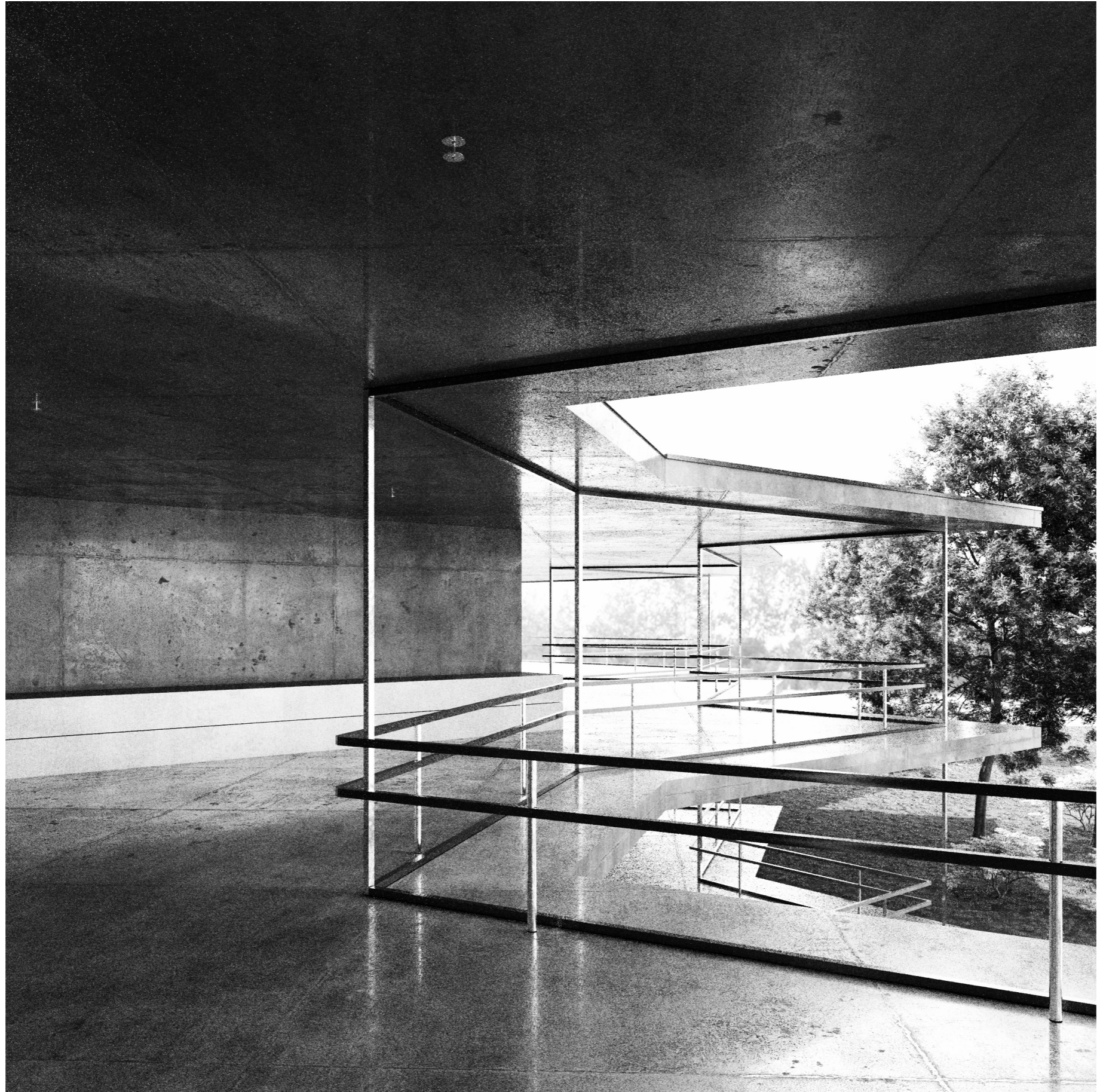
Illustration of early project in concrete
