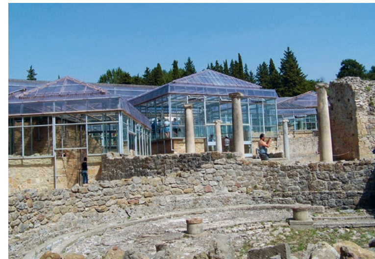
3 Protective structures designed by Franco Minissi in 1957 over the foundations and mosaic floors of the Casale villa (4th century CE) in Piazza Armenina, Sicily.
