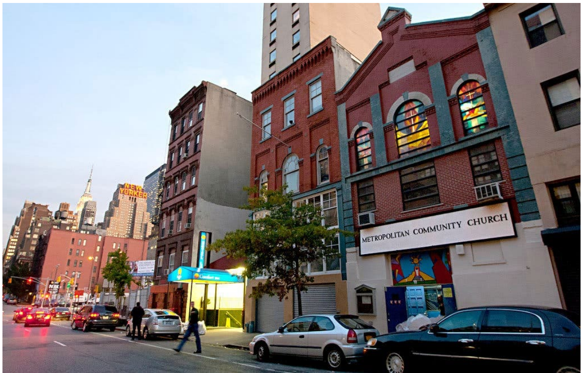
WEST 36TH Metropolitan Community Church houses a shelter.
