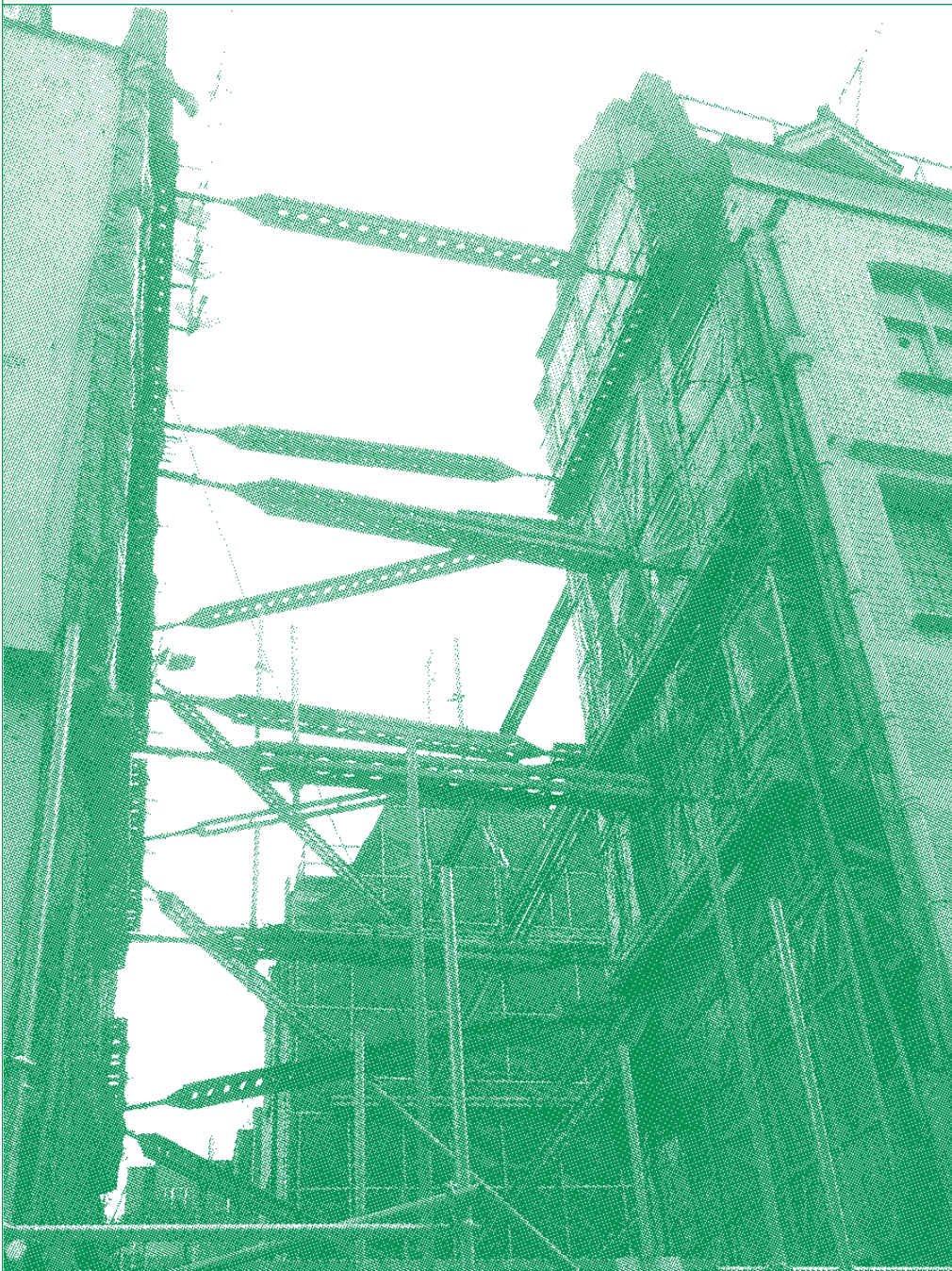
a study into scaffolding: scaffold survey
