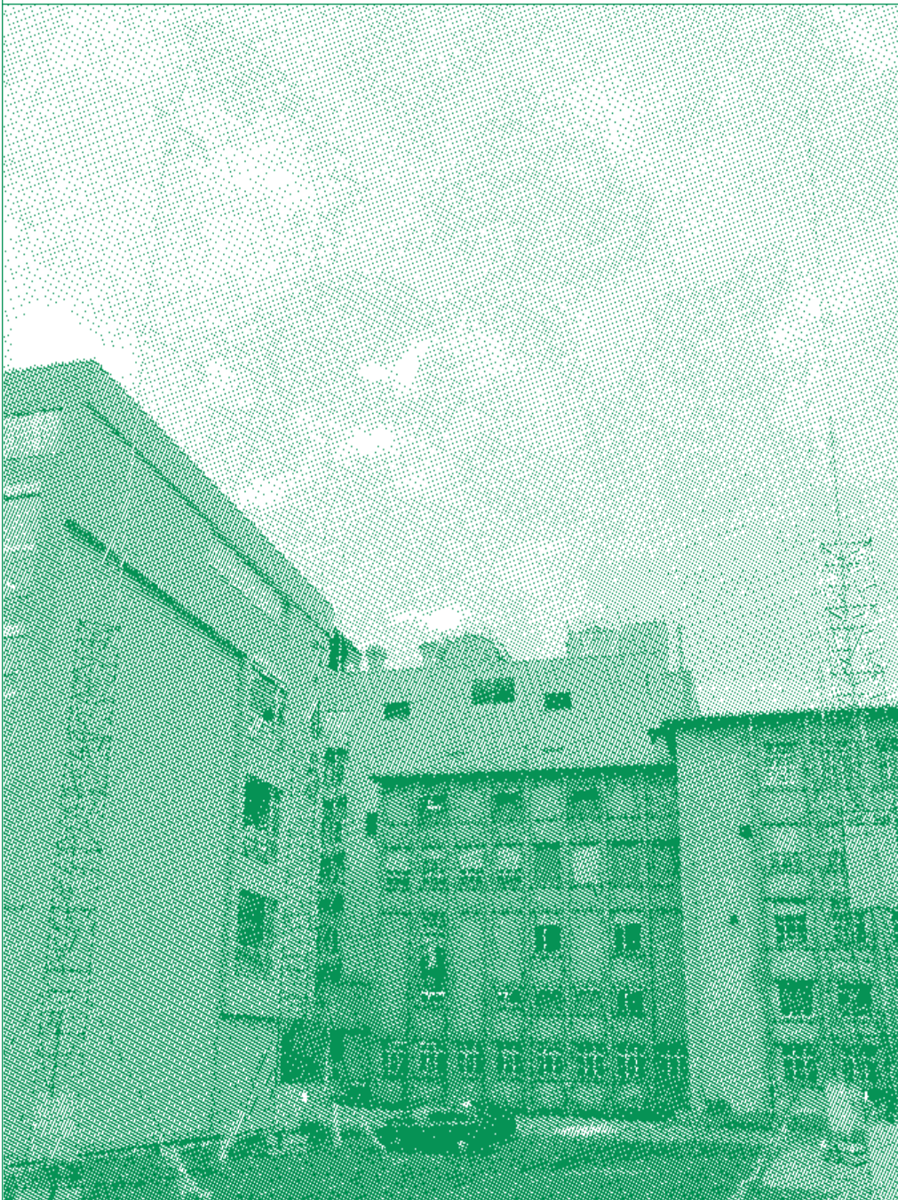
a study into scaffolding: scaffold survey
