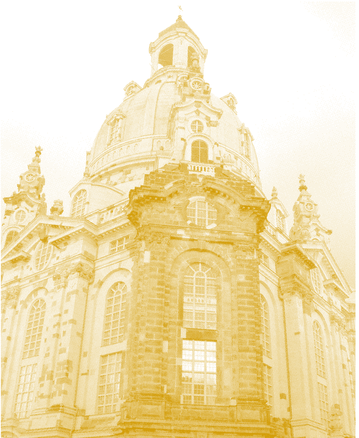
North side of Dresden Frauenkirche, showing the surviving structure and reconstruction that integrates salvaged material with in their original positions.
