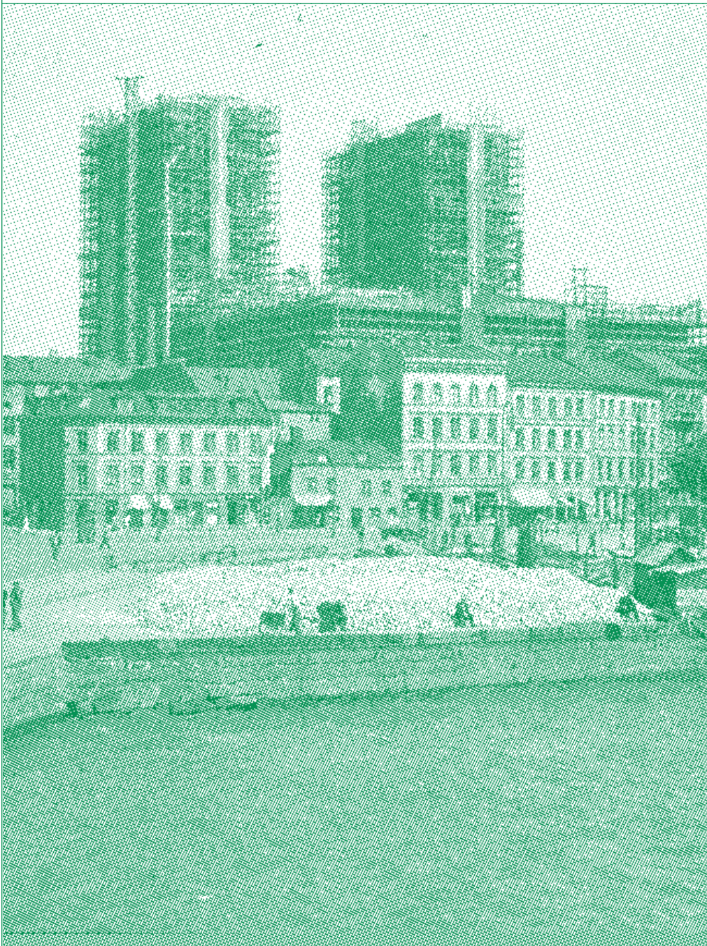
a study into scaffolding: scaffold survey
