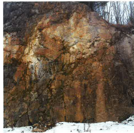
VESTVEGGEN Diagonal WEATHERING
