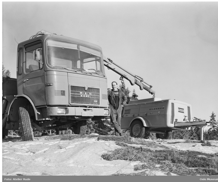
Historical photos in Huken or related to Huken. It reveals the history Huken of man power and that Huken always have been a part of a bigger urban metabolism by extracting, receiving and transforming material.
