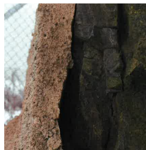
Security first. Concrete as been sprayed on some of the rock side to avoid rockslides. It serves as protection, however conceal deep pasts event.
