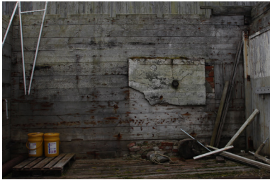
Lafted timber wall used as, insulation, interior and wind bracing
