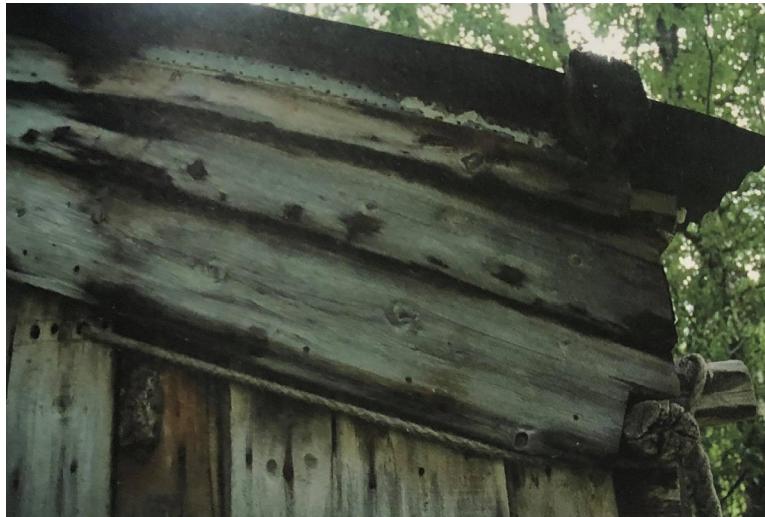
Sommerfjøs, Mellomjord. Photo: Randi Sjølie/Sametinget Picture of a summer-barn in Lyngen with cladding of reused boat strakes. 2
