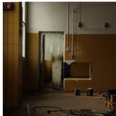
left, lost, broken
