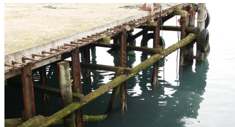
Existing pier, with 2x2 m grided foundation
