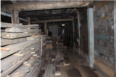
Wooden materials used for the frame, stored at site today
