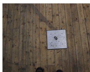
Hole in the floor for washing
