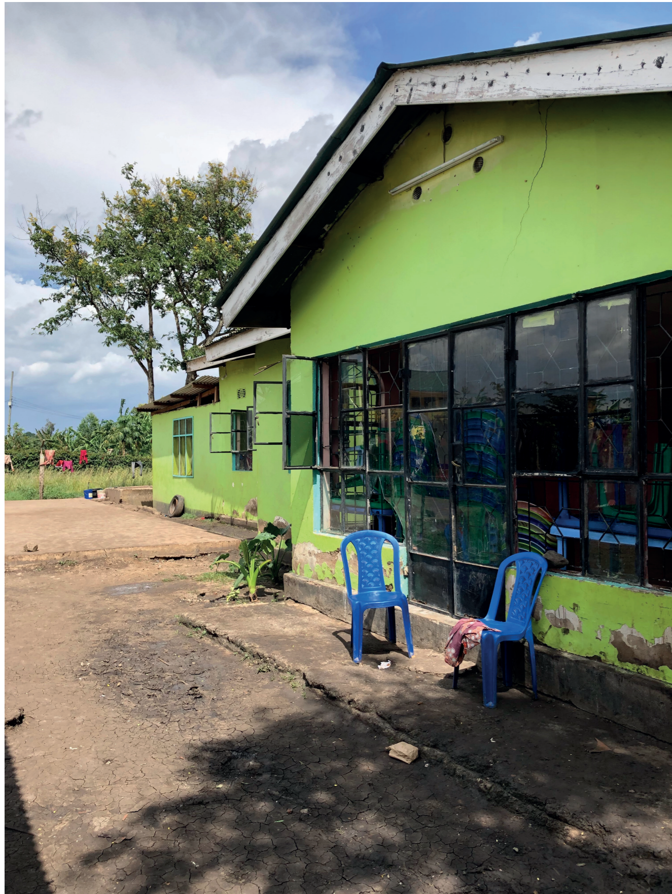
FIGURE 13: Orphanage building, windows to the classroom/playroom
