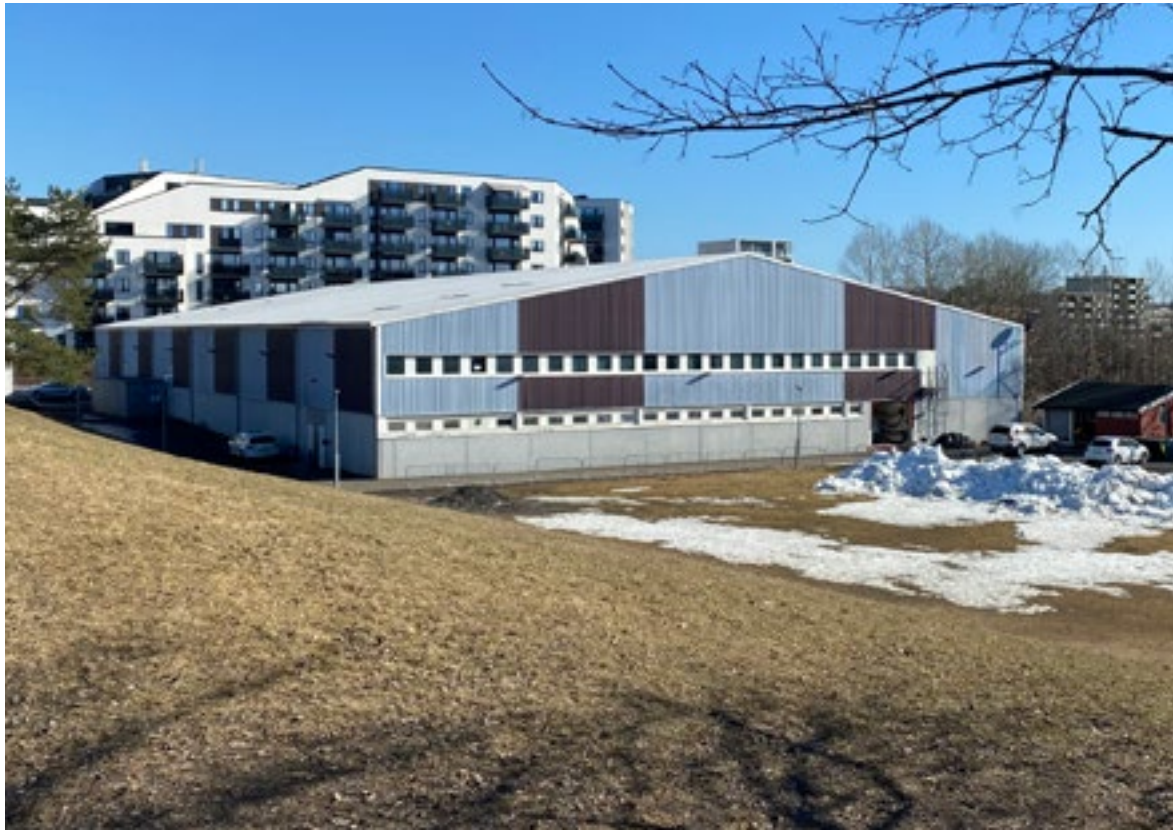
Fig. 6. Photo: Facade, west and north.
