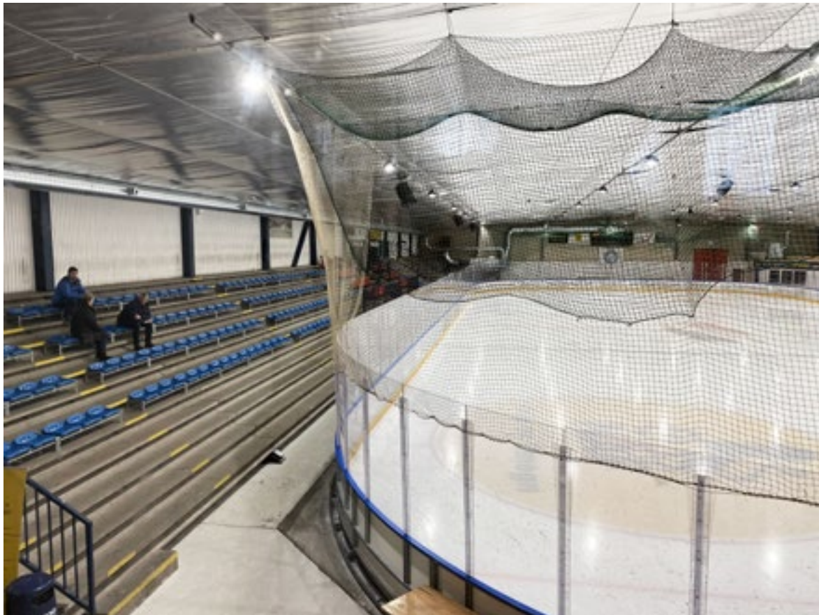
Fig. 7. Photo: Interior, ice rink and grandstands.
