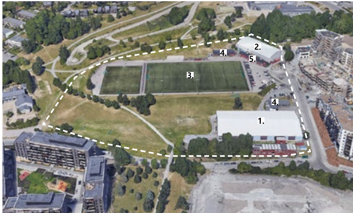
Fig. 1. Overview photo, structure presentation
