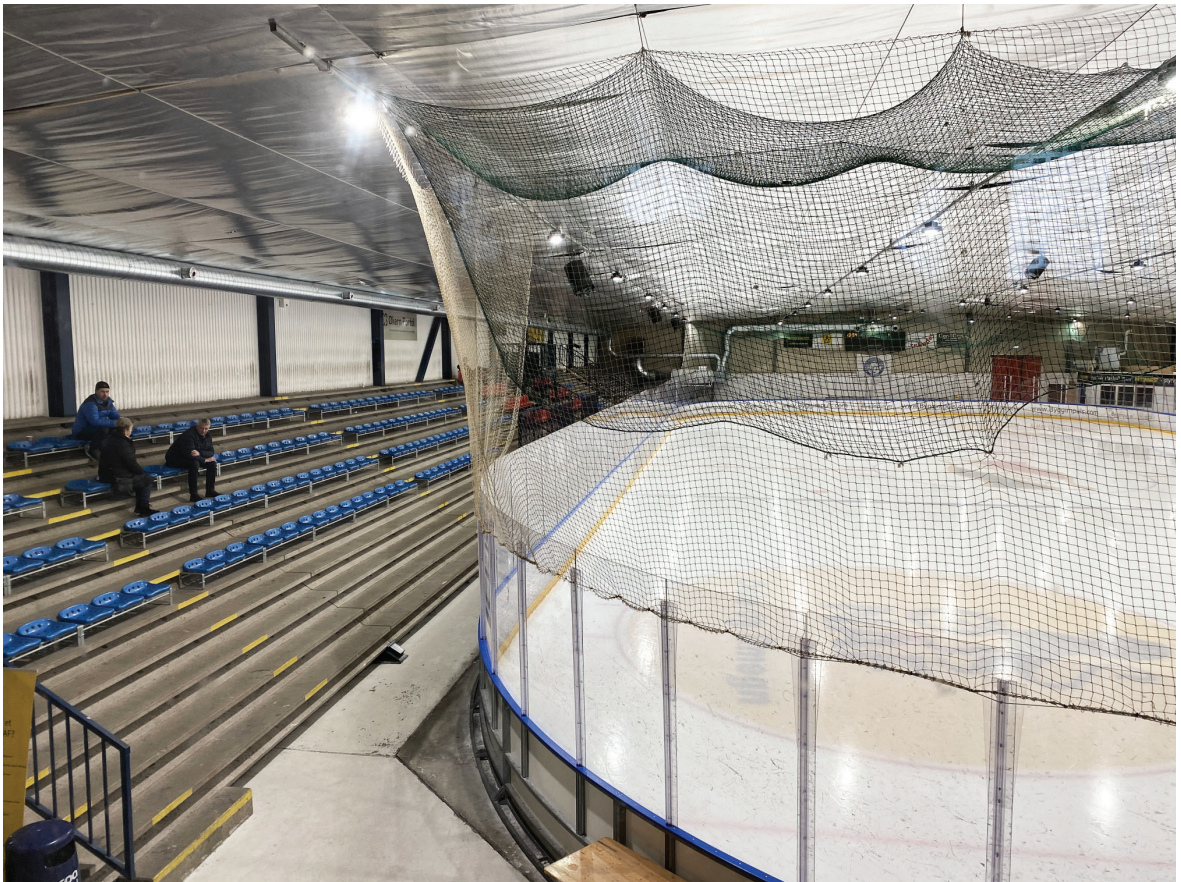
Fig. 5. Photo: Interior, ice rink and grandstands.
