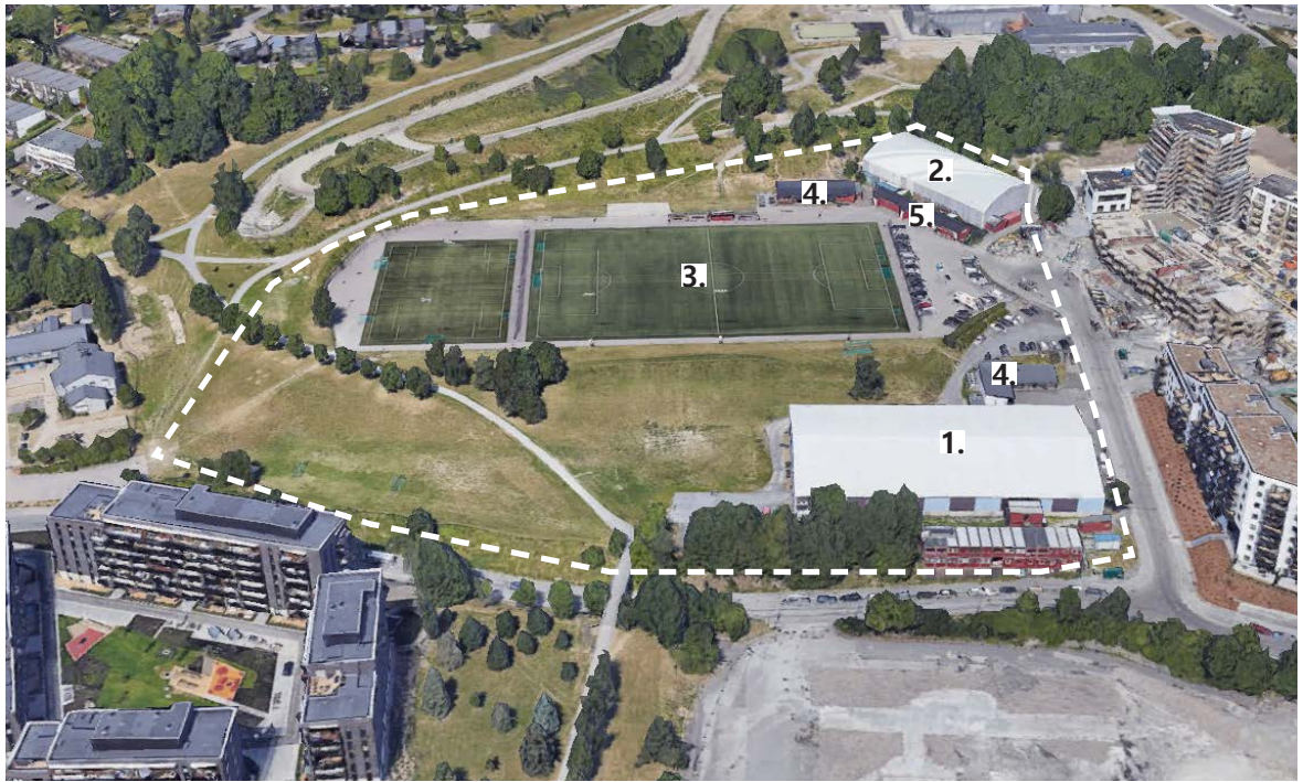
Fig. 32. Overview photo, structure presentation
