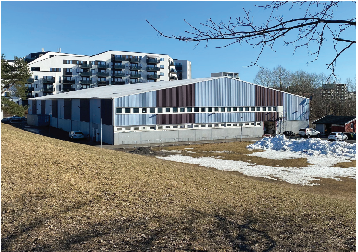
Fig. 4. Photo: Facade, west and north.
