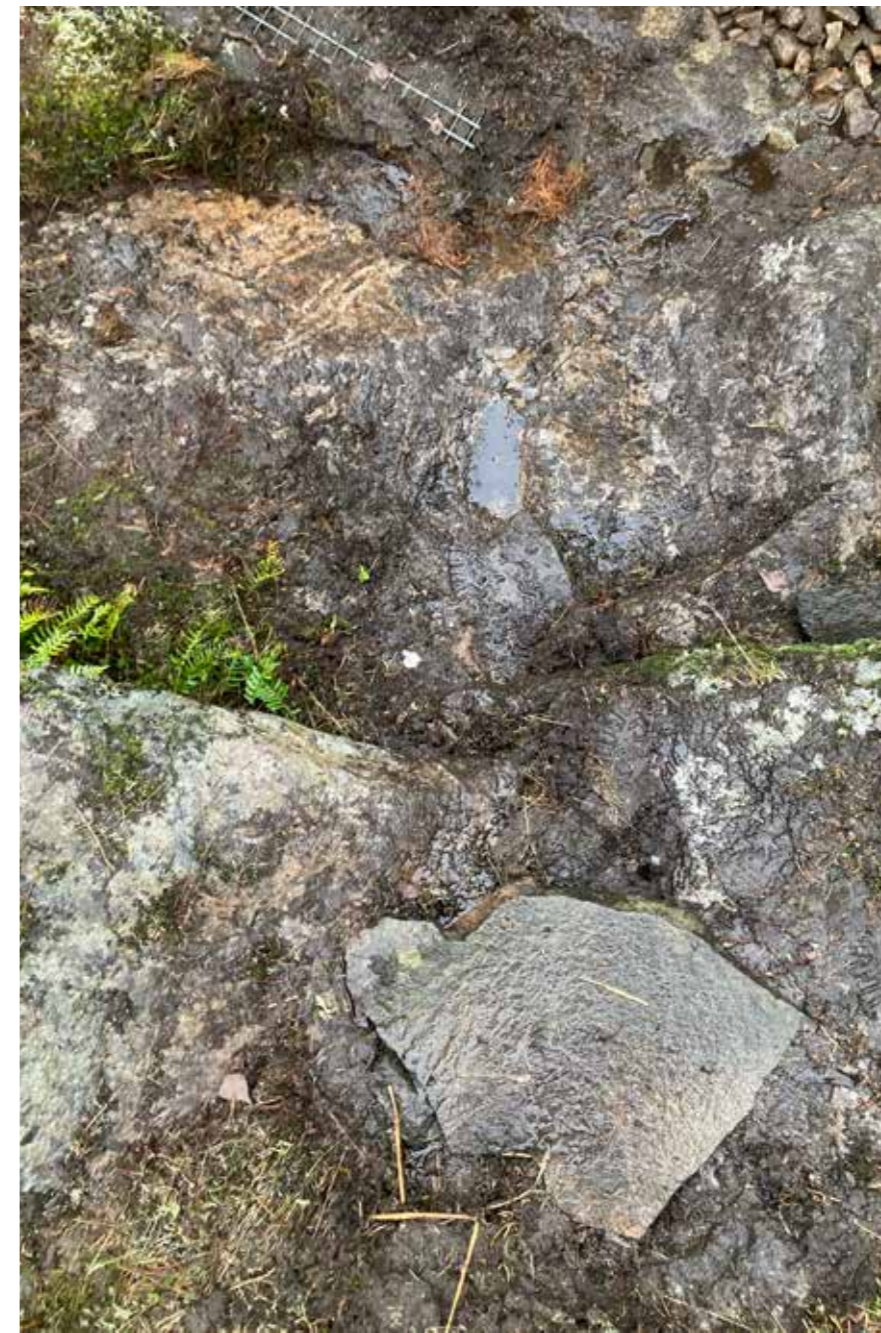
The path from the house to the utedo has been created along the way. We have added stone from clearing the site and pieces from the elephant grate as needed.
