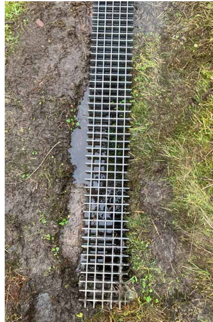
The path from the house to the utedo has been created along the way. We have added stone from clearing the site and pieces from the elephant grate as needed.
