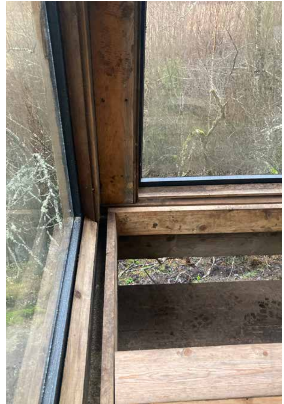
Tracks for planned screens to be pushed back and forth on wheels. To regulate visibility/sun.
