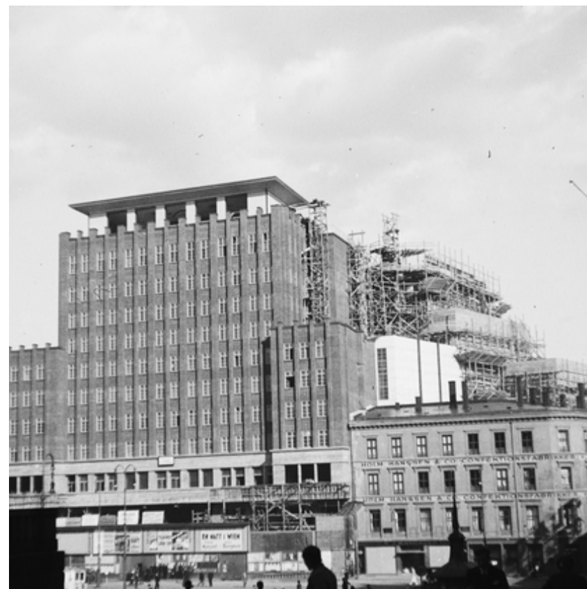
Framework to Youngstorget 2 finished, and construction the theatre's framework 1934
