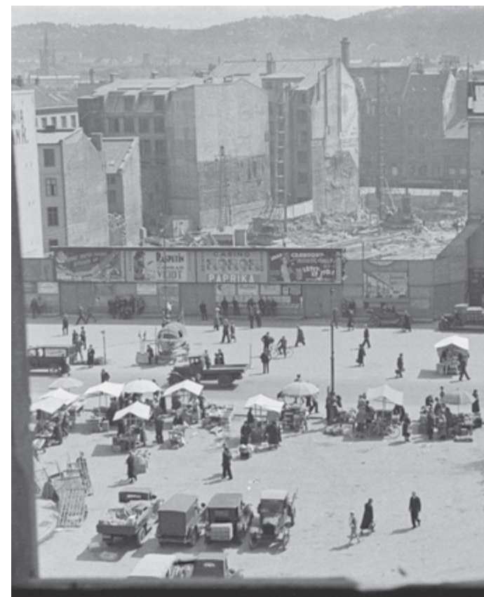
Bazarhallen and Auktionshuset demolished 1933
