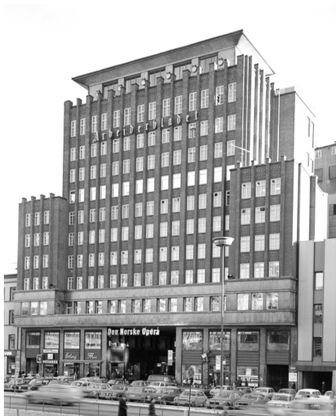
Right before new windows (3rd-11th floor) 1976
