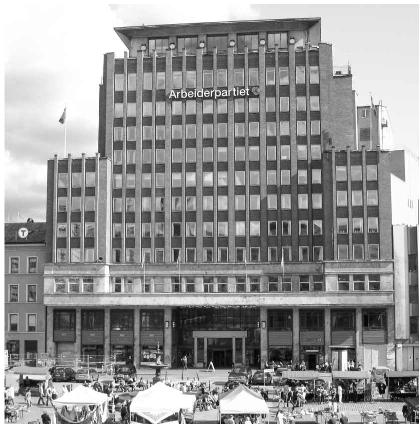
The facade's commercial profile 2003
