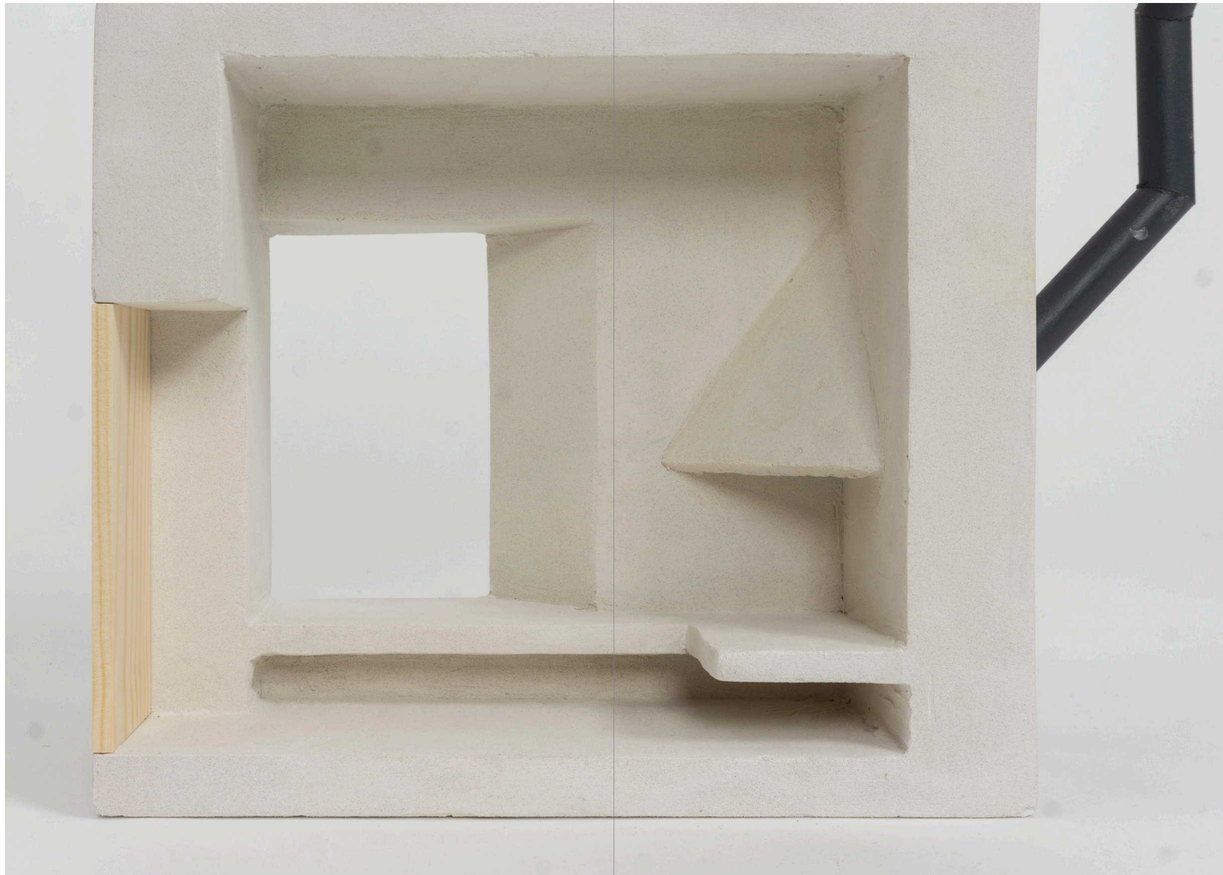
The concrete of the walls is used to create the furniture which is needed in the bedrooms.
