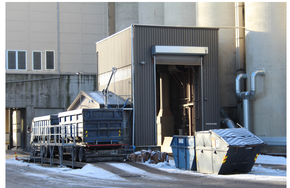
The patchwork structure of Holmen is visible both in plan and photos.
