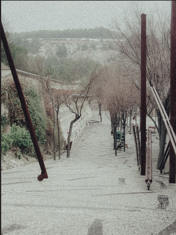
As one enters the site, one confronts a set of conical steel poles that double as gates to the cemetery – the poles are likened to the crosses at Calvary.
