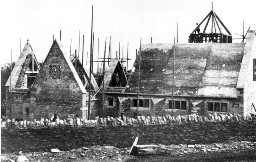
Figure 18. All Saints', Brockhampton, Construction Photograph.
