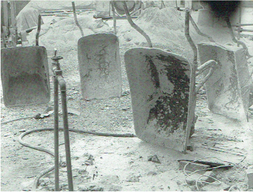
Nigel Henderson, Construction site in Hunstanton. 1953.
