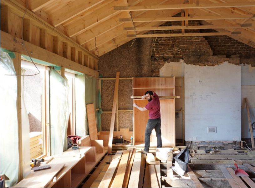
Figure 3. Building Site, Clapton House, London, Hugh Strange Architects. 2015. (Photo: Hugh Strange)
