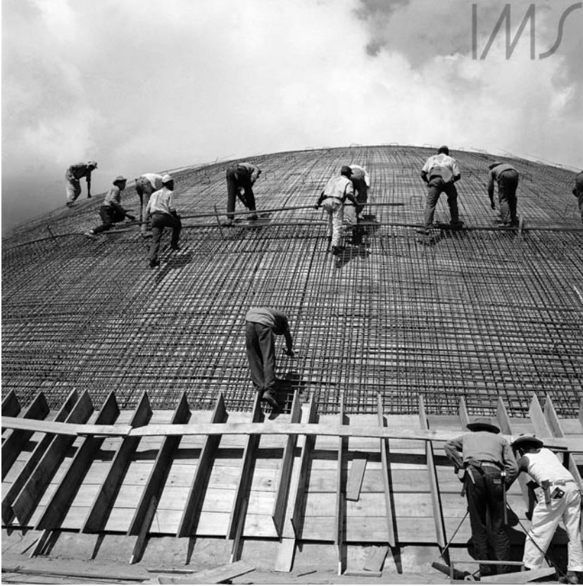
Figure 11. Brasilia construction workers as described by Sérgio Ferro. (Photo: Marcel Gautherot)
