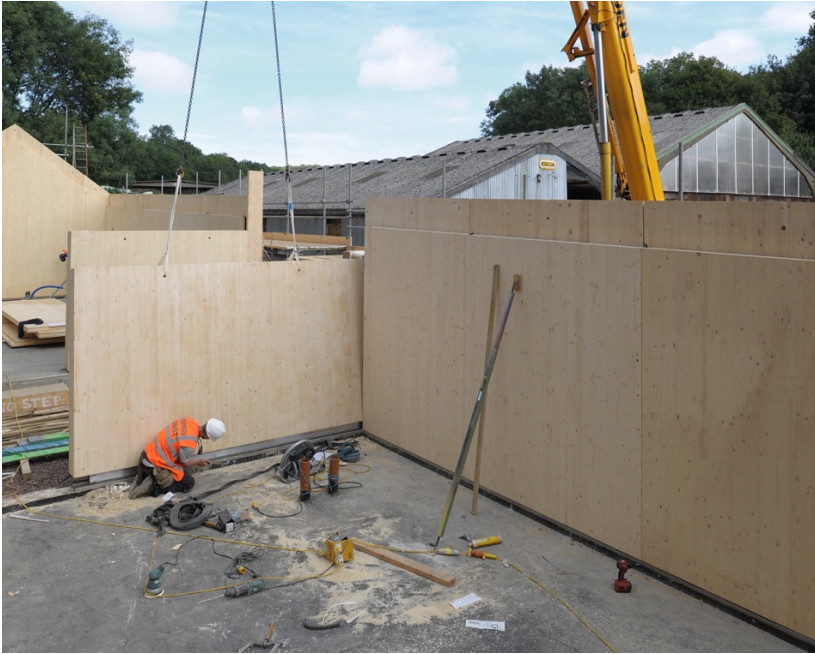
Figure 2. Building Site, Drawing Matter, Somerset, Hugh Strange Architects. 2014. (Photo: David Grandorge)
