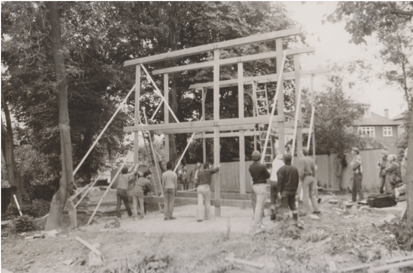
Figure 24. Walter's Way, Raising the frames. (Photo: Jon Broome )
