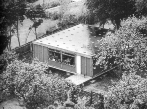
Figure 4. Highgate temporary house.
