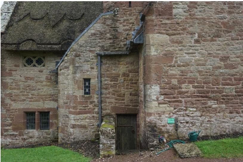
Figure 17. All Saints', Brockhampton, Expressive drainage detailed, undrawn. (Photo: Hugh Strange, 2019)
