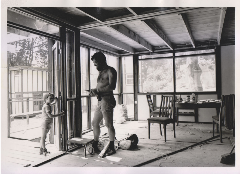
Figure 23. Walter's Way, Site Works. (Photo: Jon Broome)
