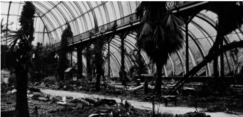
Figure 19. The Decayed state of the Great Stove, Chatsworth prior to demolition (1910's).
